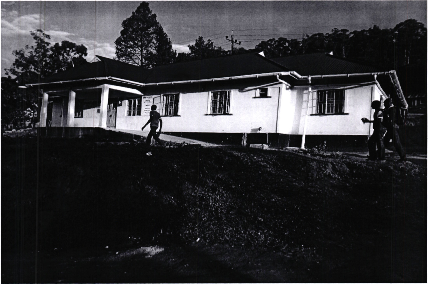
Figure 2. Komotobo Secondary school Administration Block Completed in Fy 2018/2019
