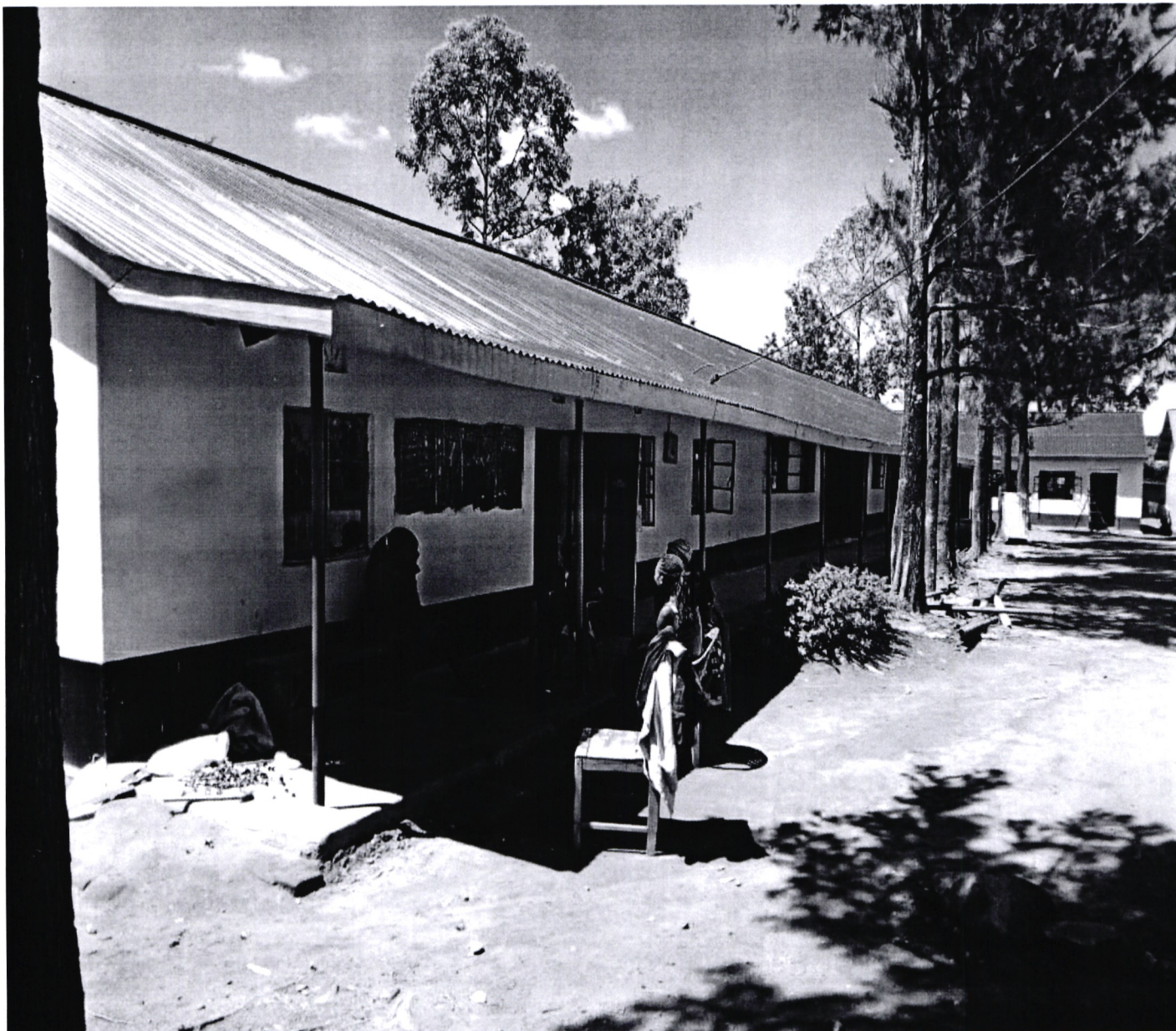
Figure 3. Nyankongo Primary .Renovation of nine classrooms and Administration Block
