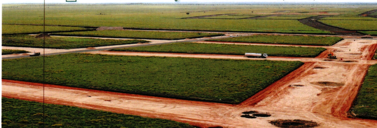
Aerial view of phase 1 Horizontal infrastructure
