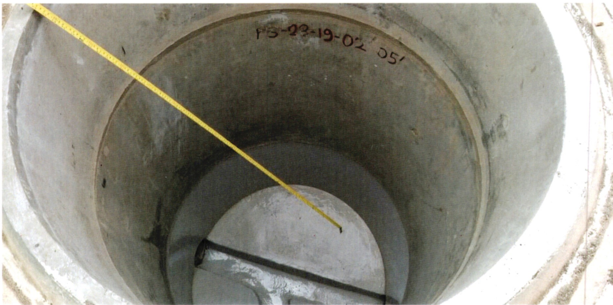
A section of WRP under Constructions
