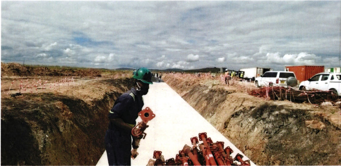
A section of utility tunnel under construction
