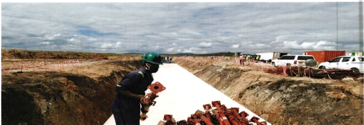
A section of utility tunnel under construction
