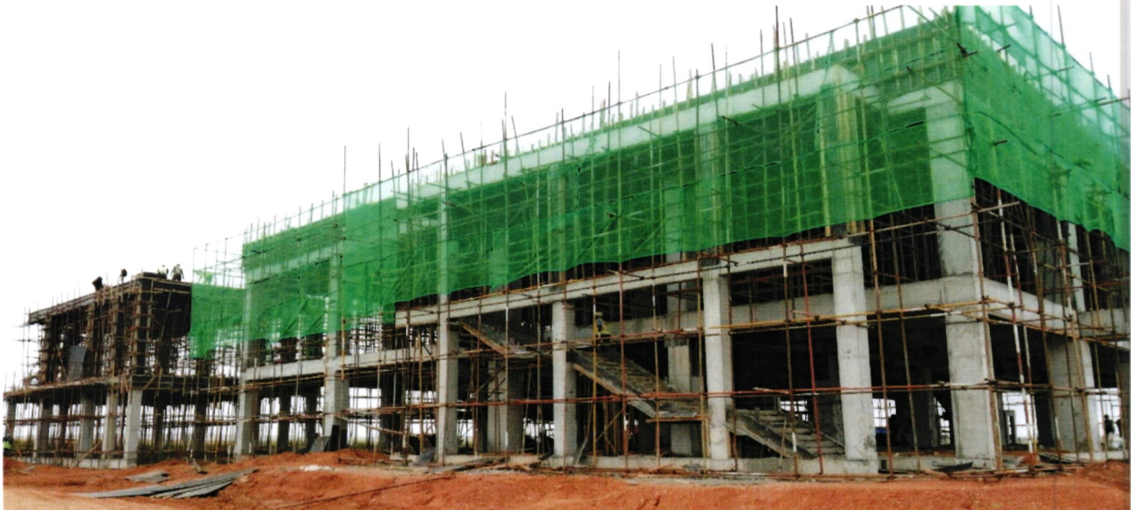
Civil works for the primary Data Centre
