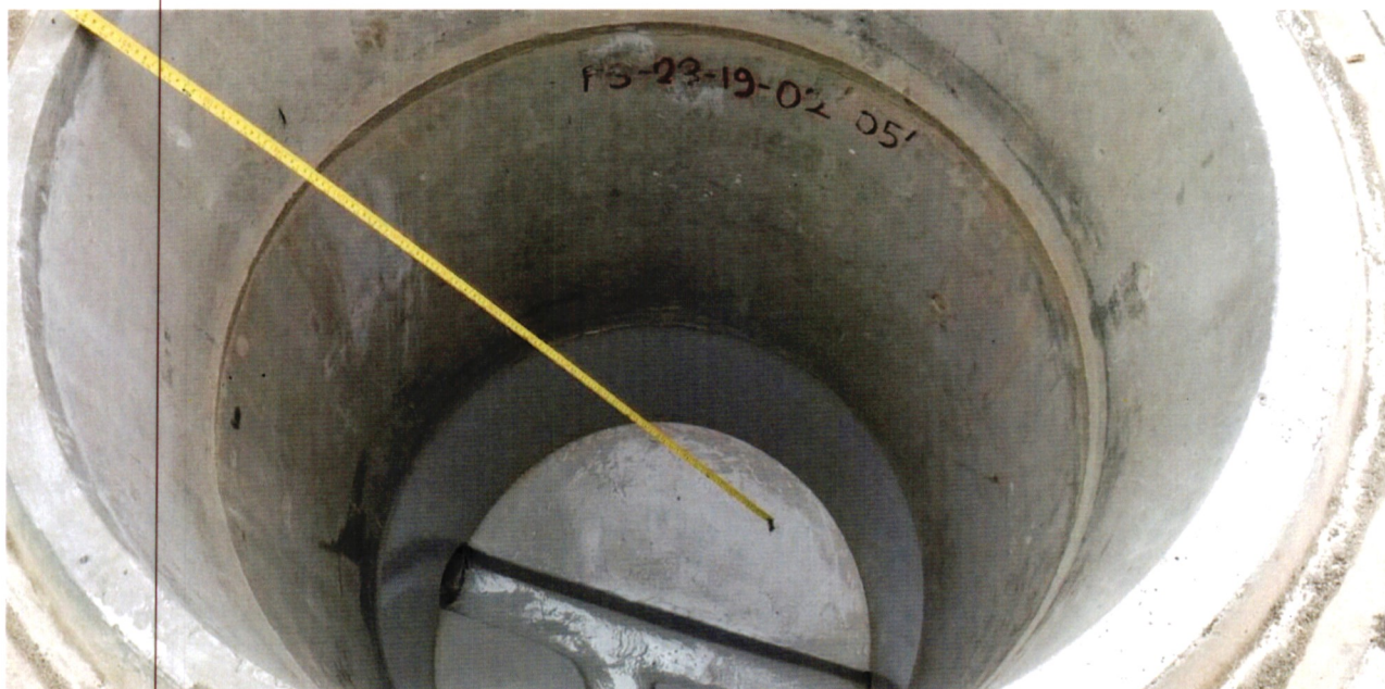
A section of WRP under Constructions
