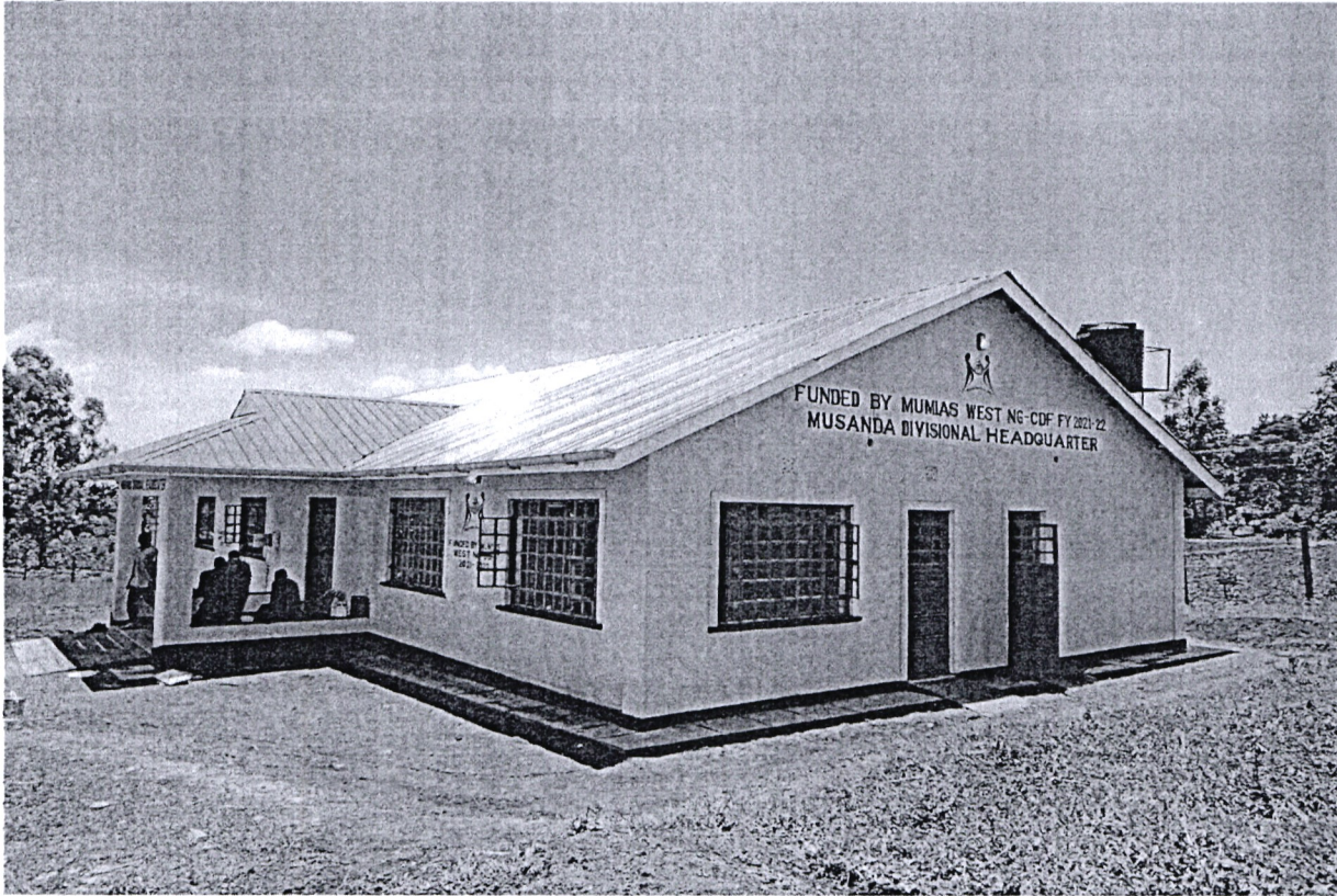
Musanda Divisional Headquarter- Construction of Administration Block
