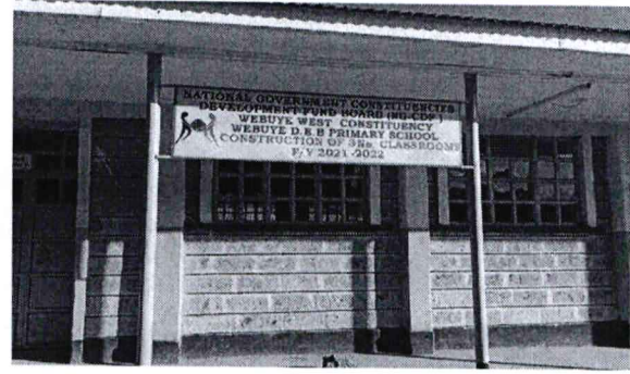
Webuye D.E.B Primary school Classrooms
