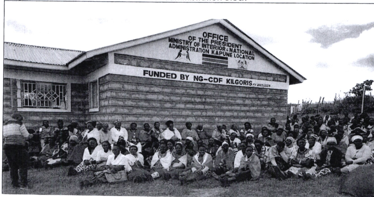
Kapune chief's office - construction of administration block
