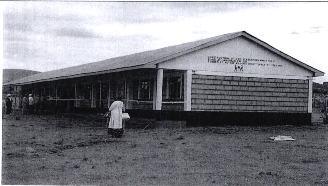
OLAMURIAKI PRIMARY SCHOOL – Construction of classrooms
