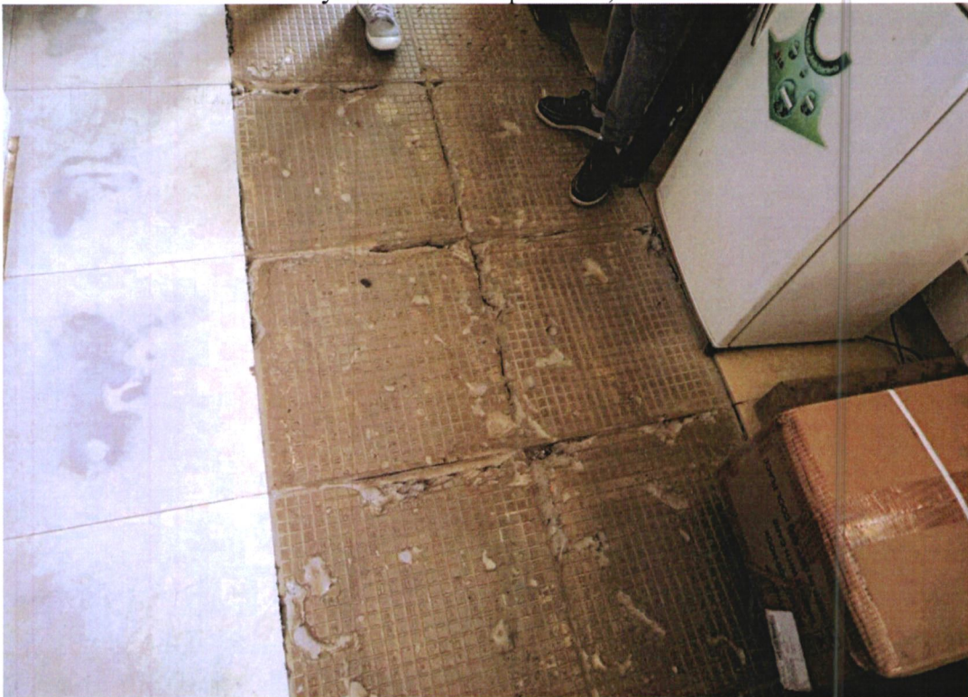
Picture 2: The cracked floor at the main corridors and common areas of the Bungoma County Referral Hospital.
