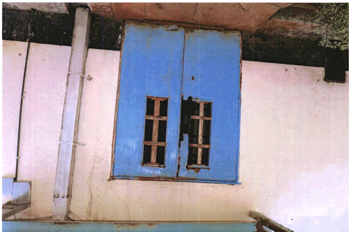
Picture 28: The deteriorated state of infrastructure at Kakamega County Referral Hospital, exemplified by weathered and damaged entry doors.
