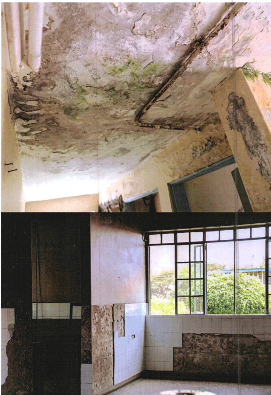
Picture 5 & 6: Severely damp and mould-infested corridor ceiling with corroded exposed pipework, highlighting chronic water leakage and poor maintenance and smoke-stained kitchen wall with extensive tile loss and exposed, deteriorated plaster demonstrating longstanding neglect of basic maintenance in the kitchen.
