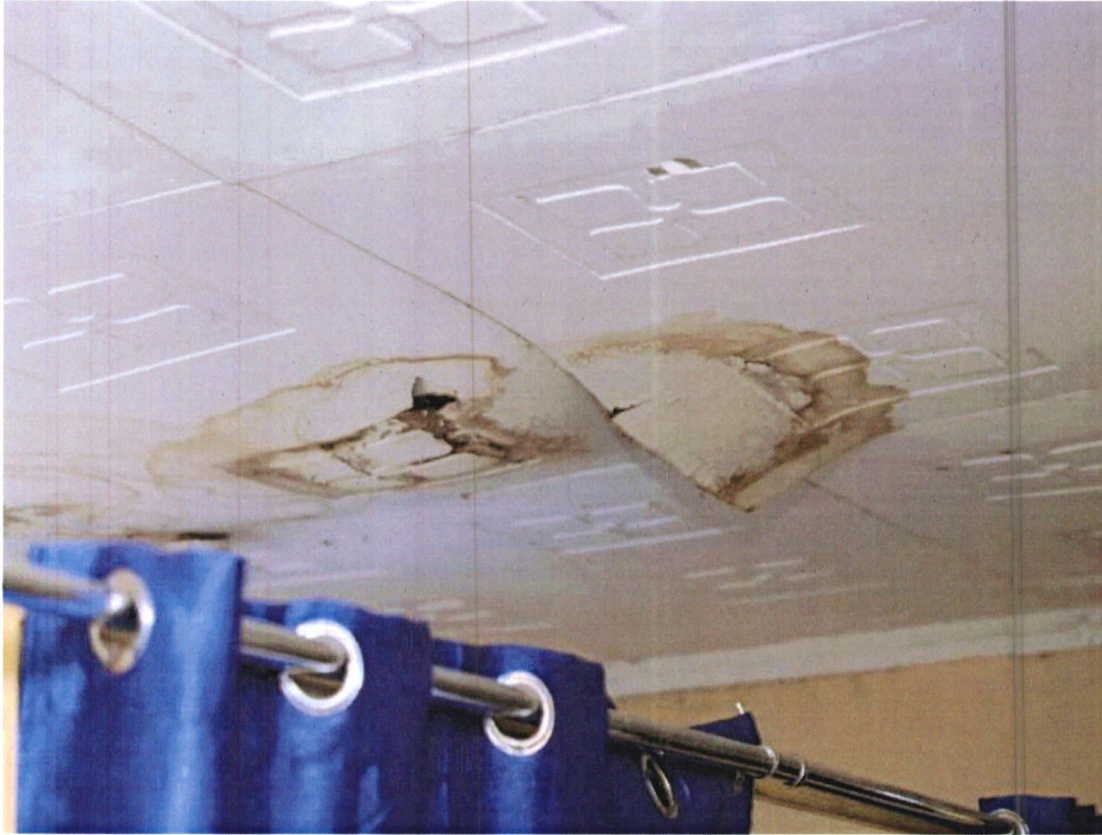
Picture 25: Ceiling damage at Kimaeti Health Centre with visible water stains, cracks and structural deterioration.
