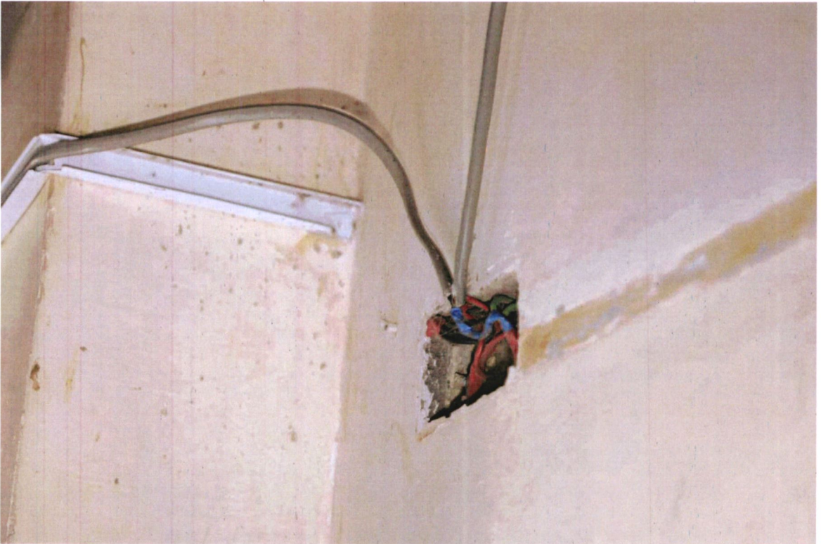
Picture 31: Exposed and poorly secured electrical wiring at Kakamega County Referral Hospital.
