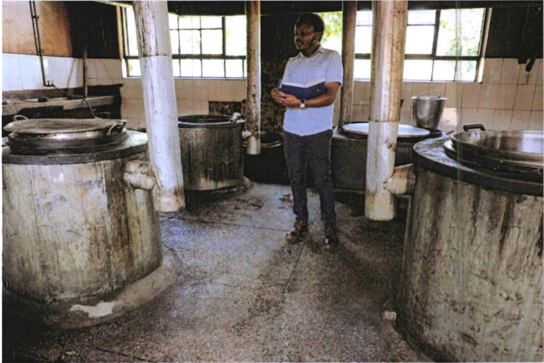
Picture 9: Old firewood-fueled hospital kitchen with large, soot-stained cooking pots and wet, slippery floor, highlighting outdated equipment and significant occupational and food-hygiene risks.
