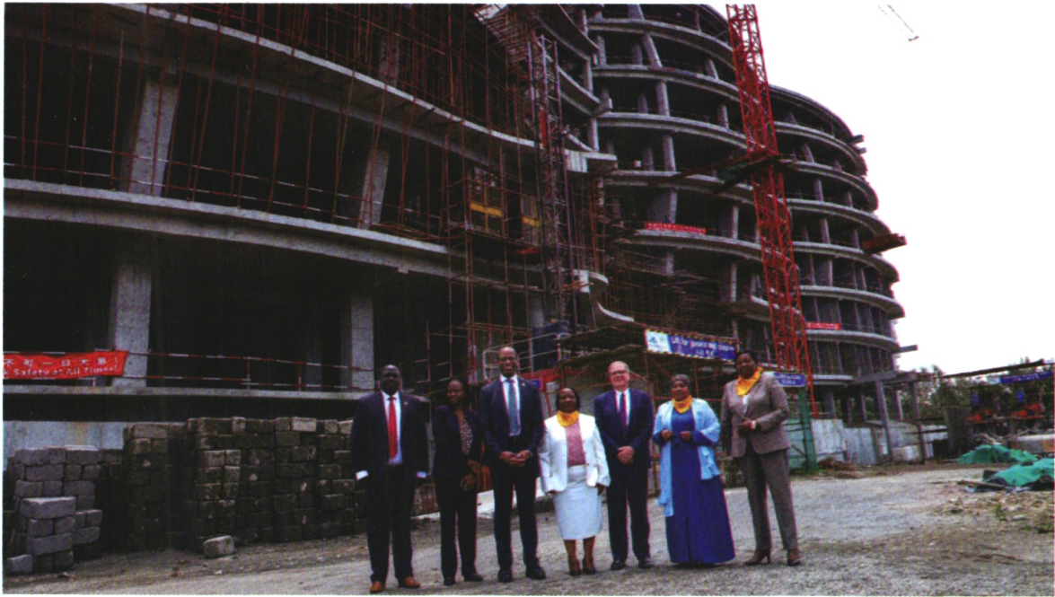
Parliamentary Service Commissioners joined by a delegation on a study tour of the Parliament of Kenya, conduct a tour of the ongoing construction of the CPST Complex in Karen.
