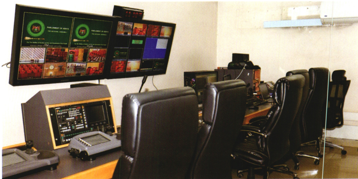
The upgraded broadcasting system prepared for digital recording using Hyperdeck technology.
