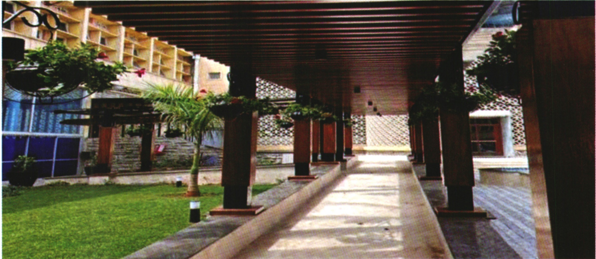
Rear walk refurbished and ramp installed for ease of access by Persons with Disabilities
