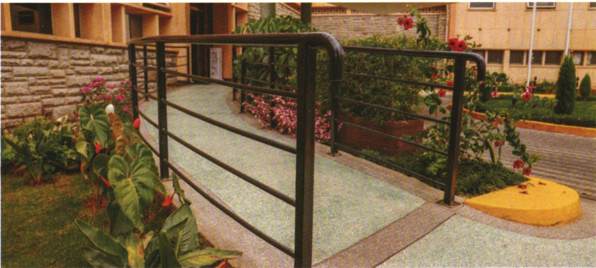
Front walkway/ramp installed to ease mobility within Parliament Buildings.
