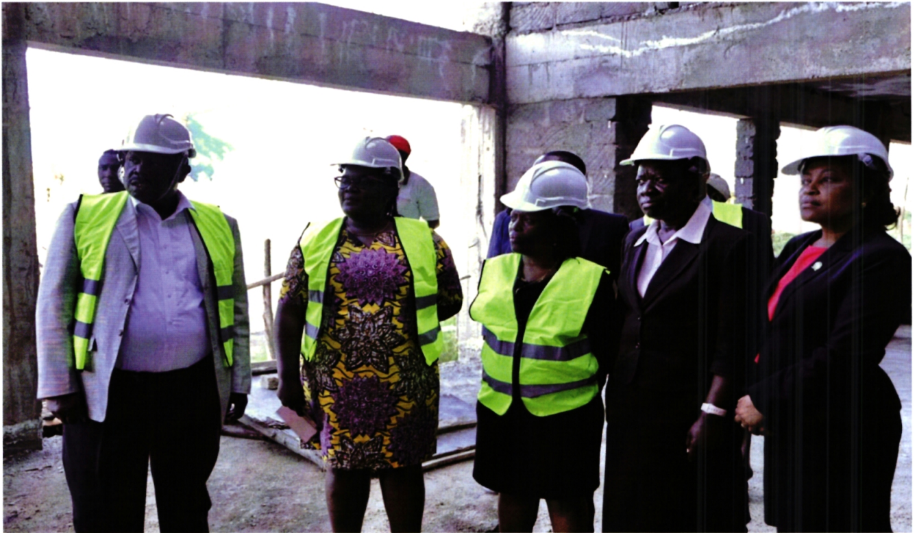
JSC Commissioners inspect ongoing construction of the Murang'a Law Courts
