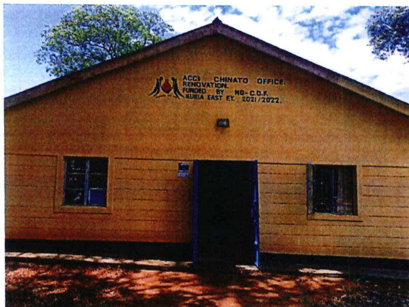
FIG 4: ACC's CHINATO OFFICE RENOVATION
