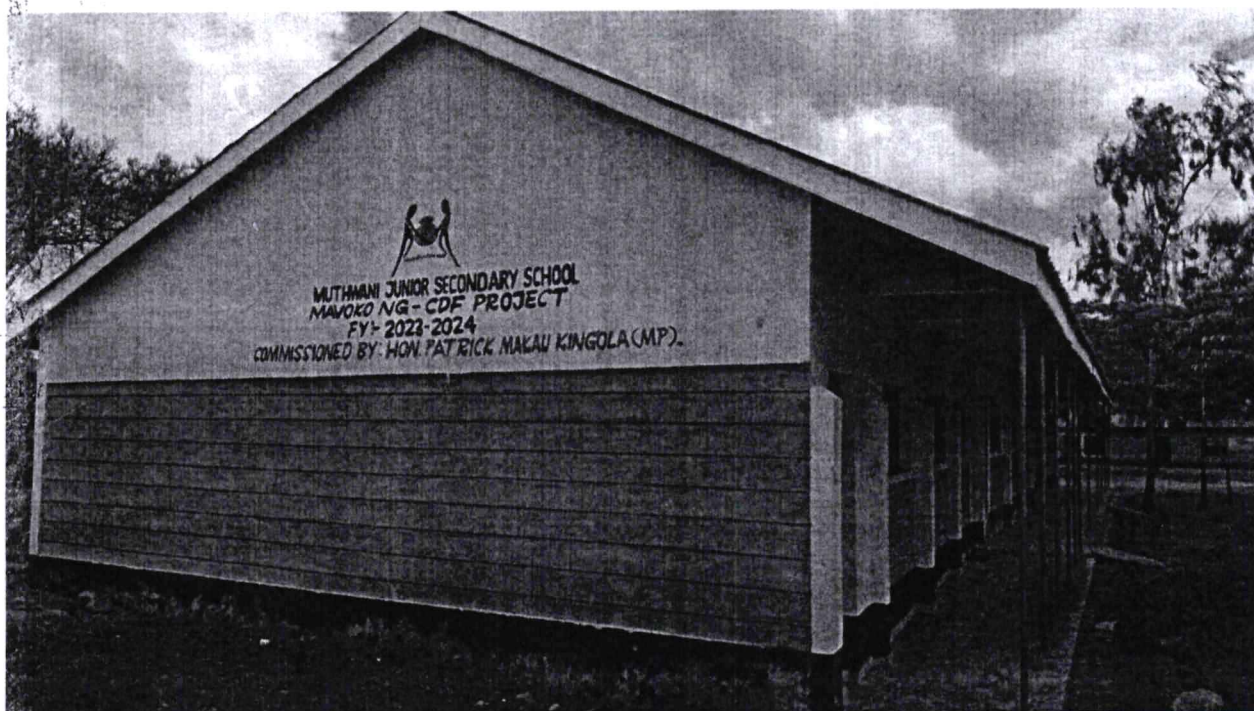
1NO. CLASSROOM BLOCK AT MUTHWANI JUNIOR SECONDARY SCHOOL.
