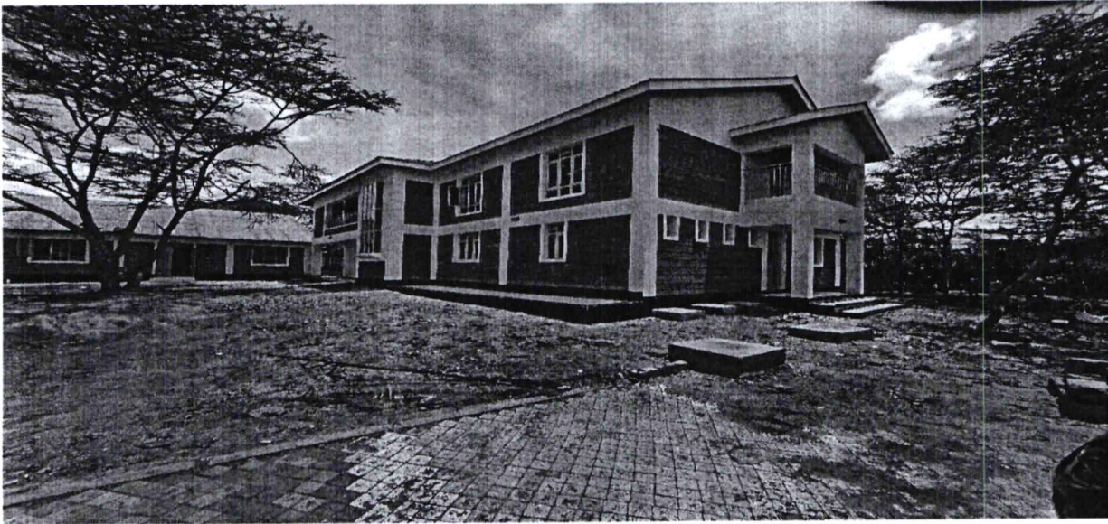
ADMINISTRATION BLOCK AT MAVOKO SECONDARY SCHOOL
