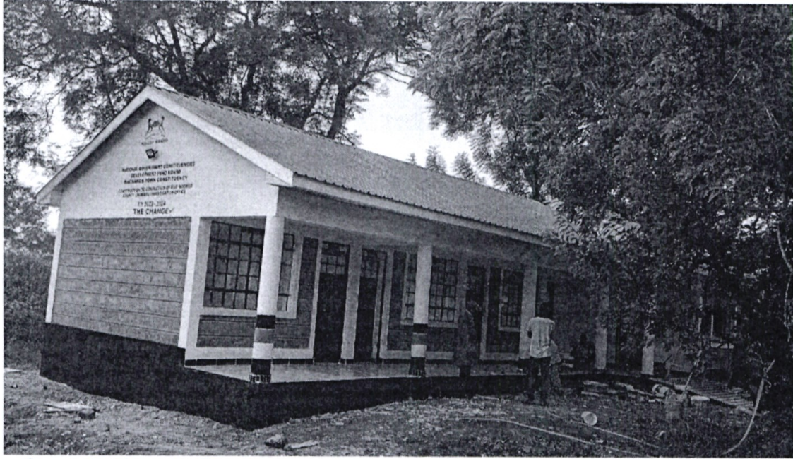
Figure 3: County Criminal Investigations Office block
