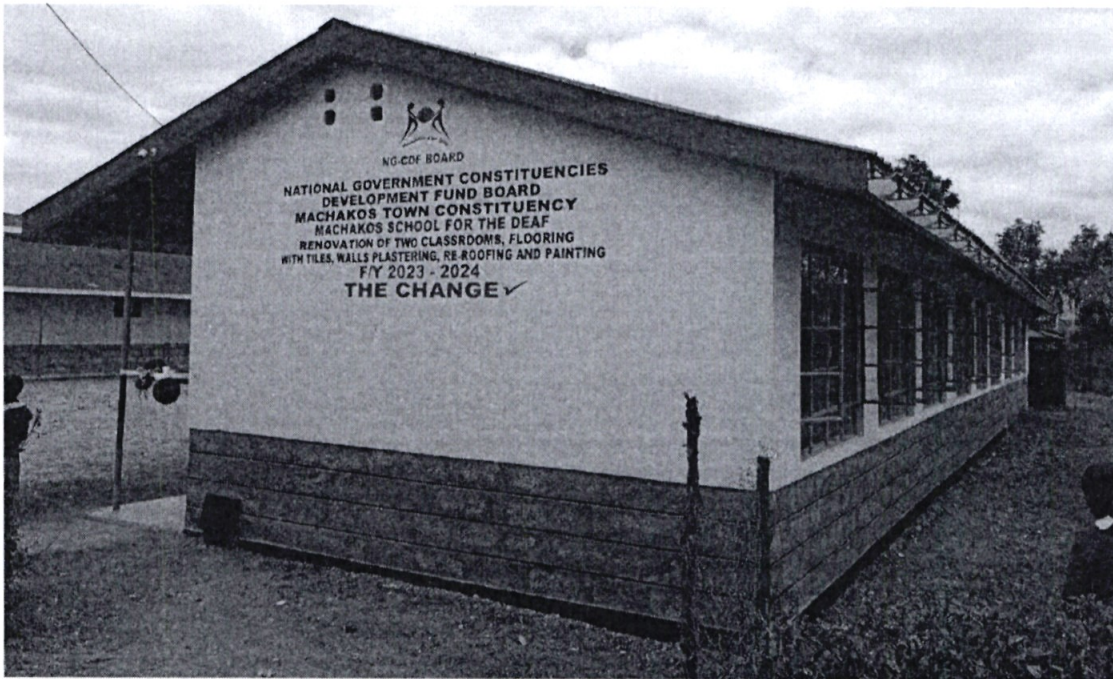
Figure 4: Machakos School for the Deaf Primary Primary School - Renovation of two Classrooms
