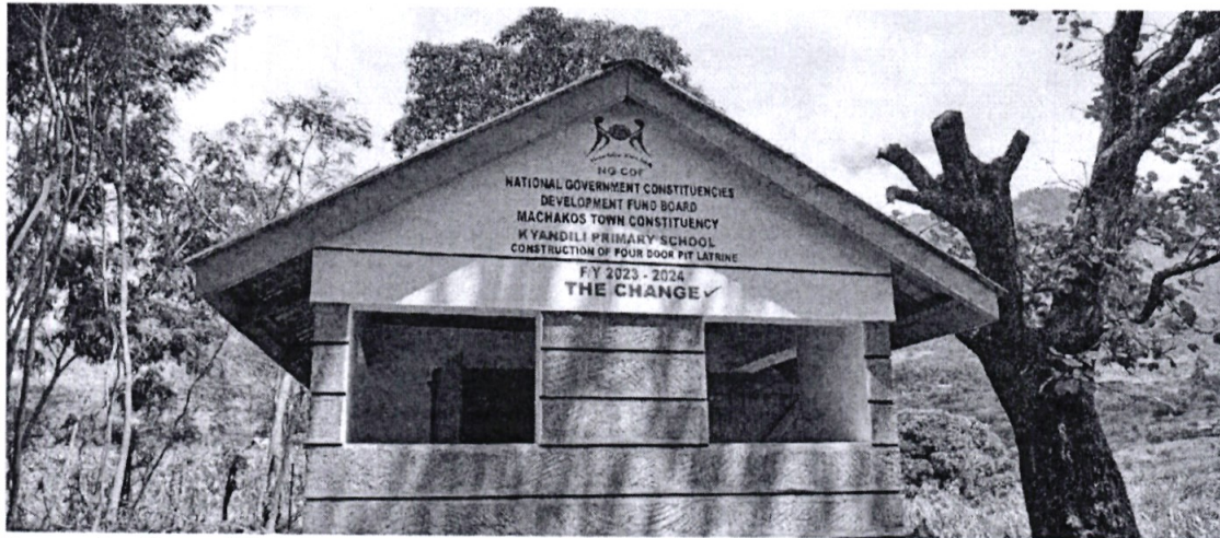
Figure 2: Kyandili Primary School 4 door Pit Latrine
