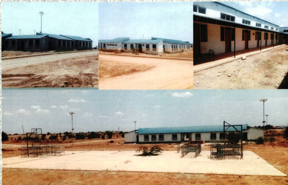
On-going construction of 2 No. Hostels
