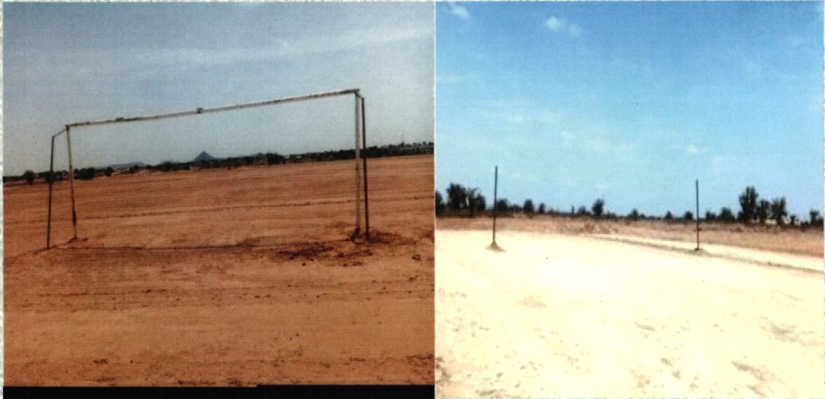
On-going construction of Sports facilities
