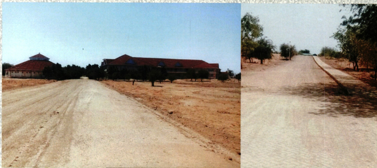
Construction of roads network at TUC
