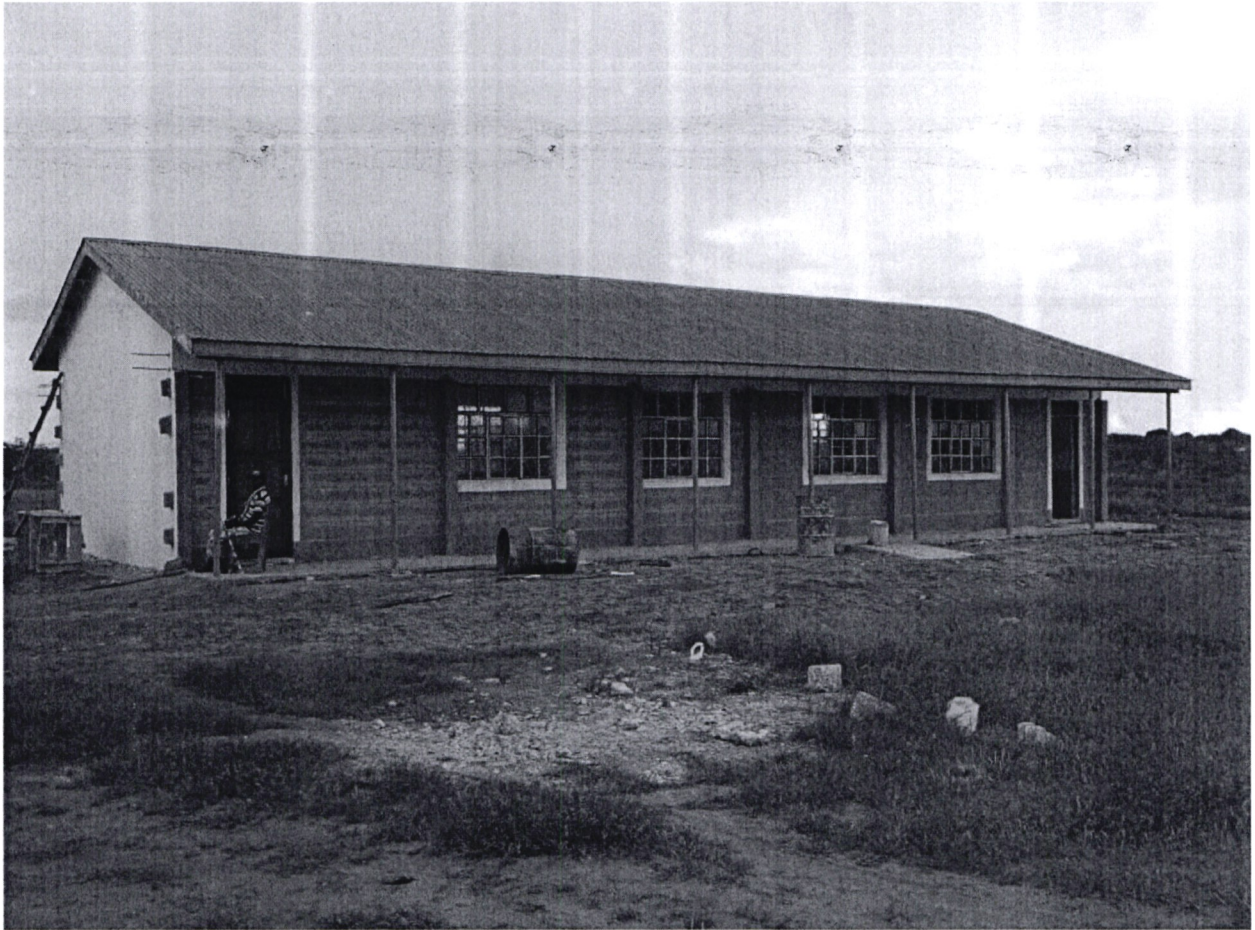
b. Construction of 2 No. complete classroom at Singwaya secondary school
