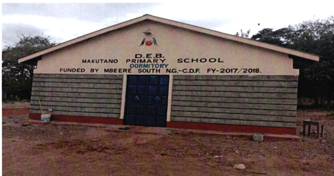
MAKUTANO PRIMARY SCHOOL DORMITORY COMPLETED LAST FINANCIAL YEAR
