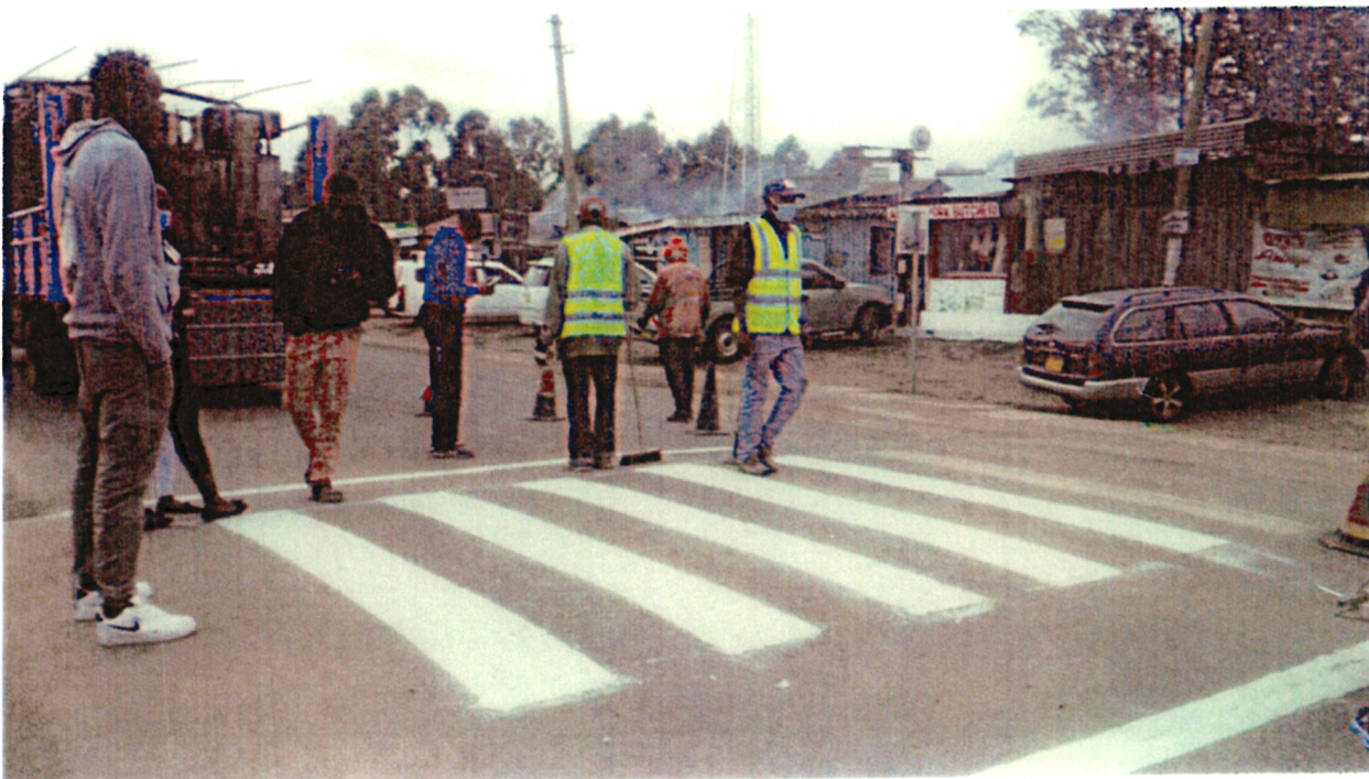
2. Ngong Kiserian: Ongoing pedestrian marking repair at 5+870
