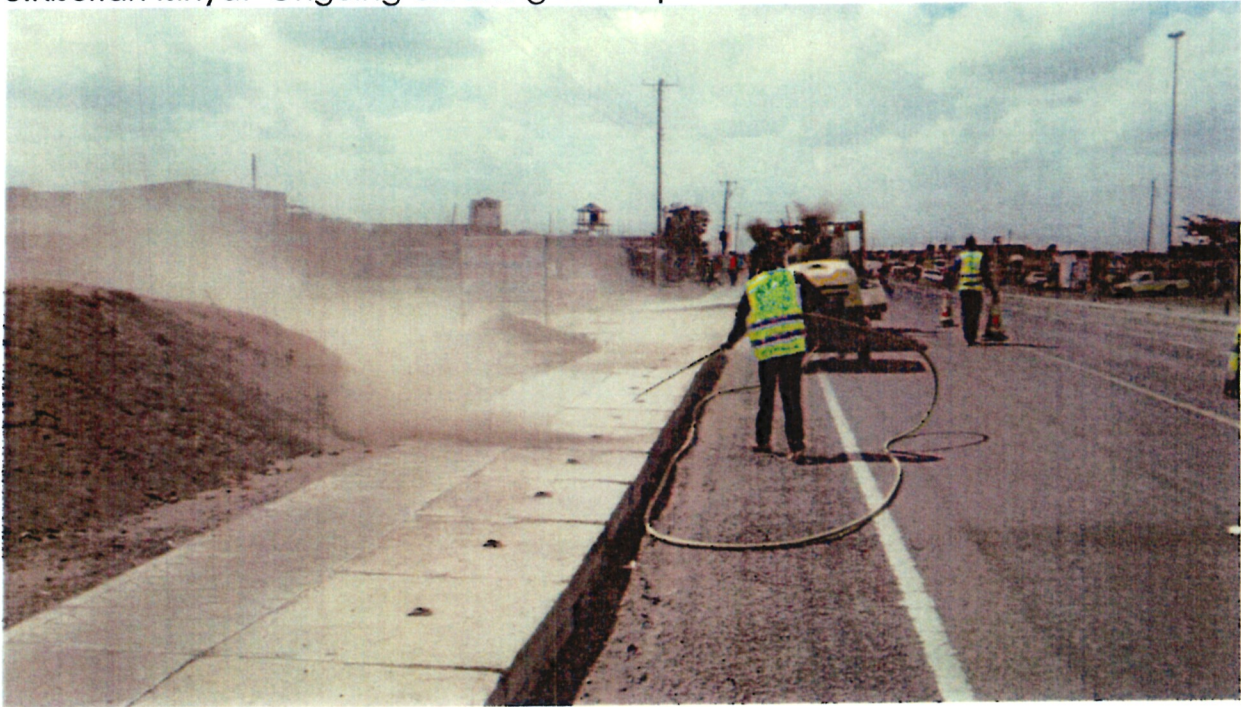
6. Kiserian Isinya: Ongoing AC repair at 29+860 RHS
