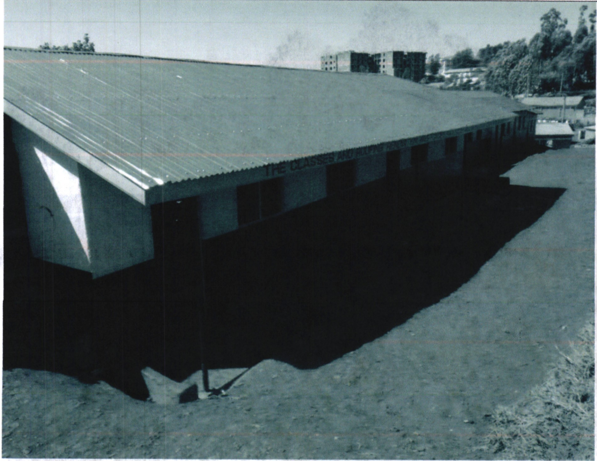
Fig 4: Renovation of 3 class rooms at Gekomu Primary School
