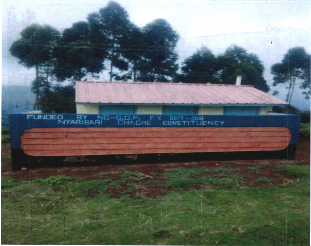
Fig 5: construction of 3 door pit latrine for girls at Kabosi Primary School
