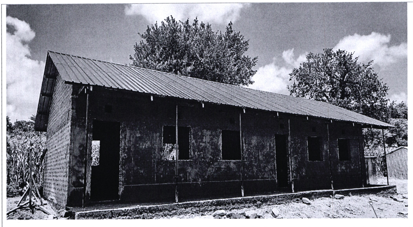
Fig. 2: Pkatieny Primary School, 2 Classrooms under Construction
