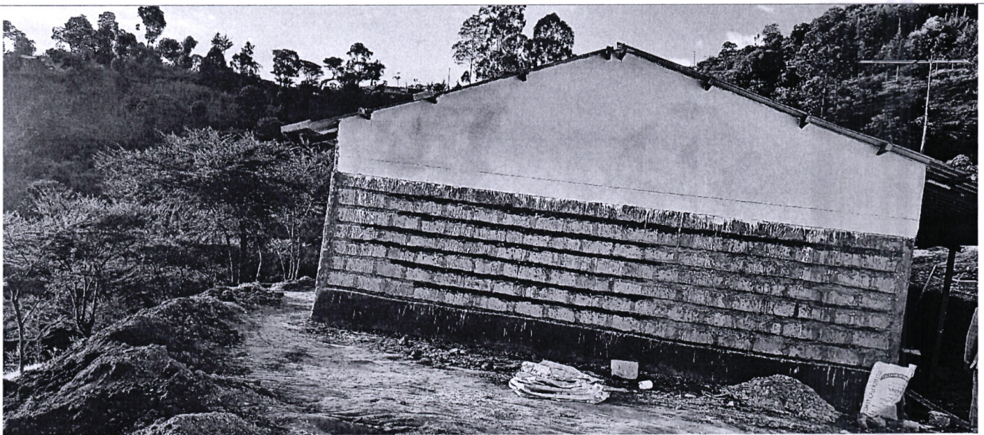
Fig. 4: E.L.C.K Chemolo Secondary school, 1 classroom under construction
