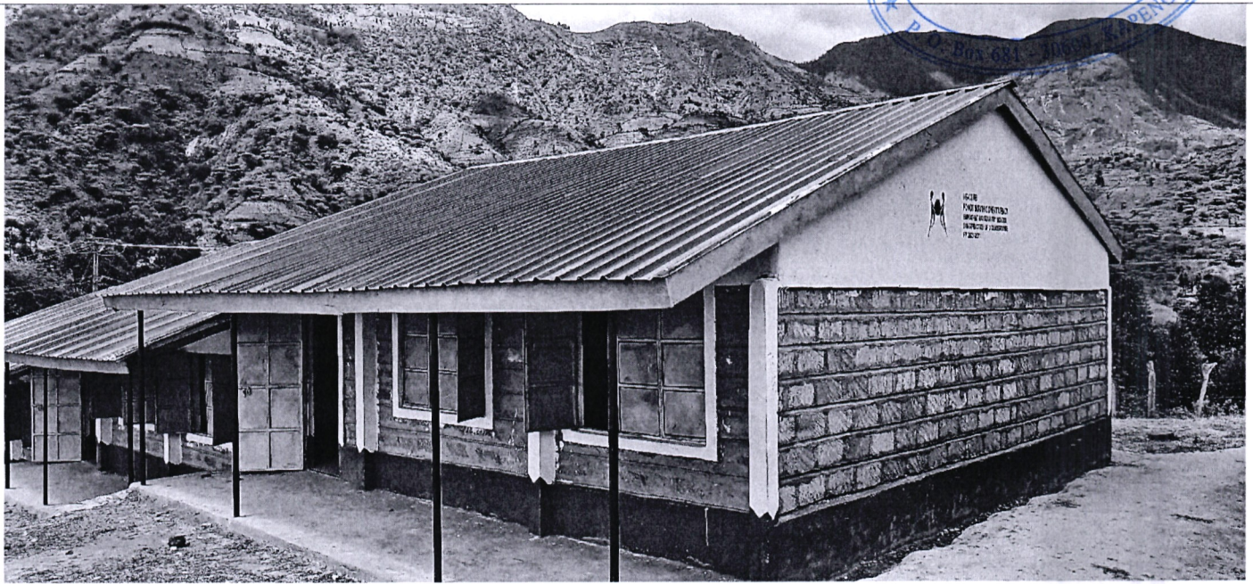
Fig. 3: Empoghat Daystar Primary School – Construction of 3 Classrooms to completion
