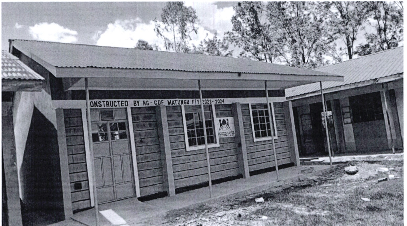
Construction of 1 Classroom at Eshibanze primary School
