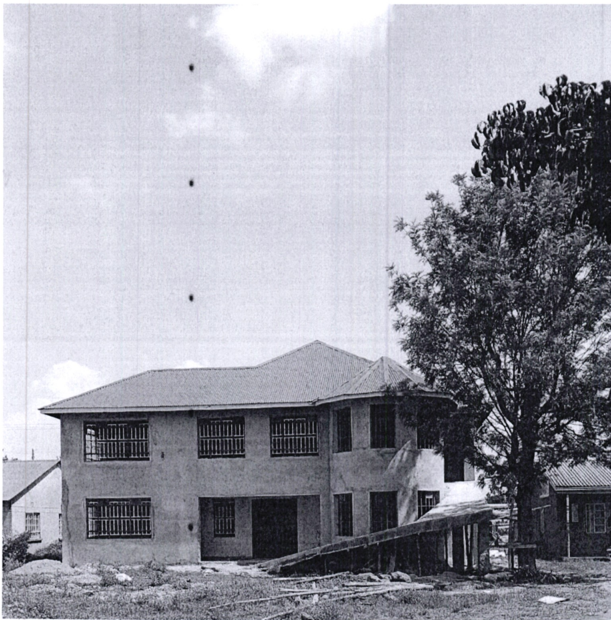
Completion of DCC office at 90 % completion
