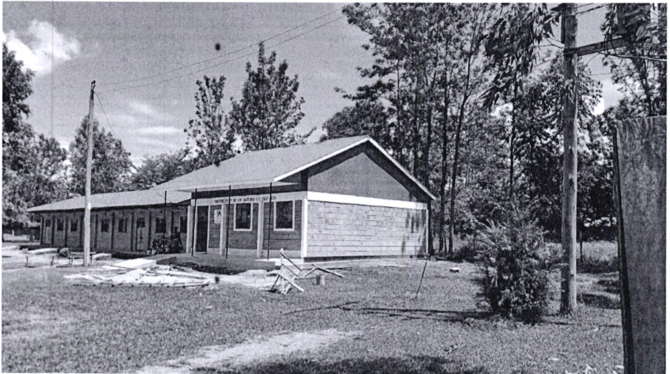
Construction of 1 Classroom at Koyonzo Special Primary School FY 2022-2023
