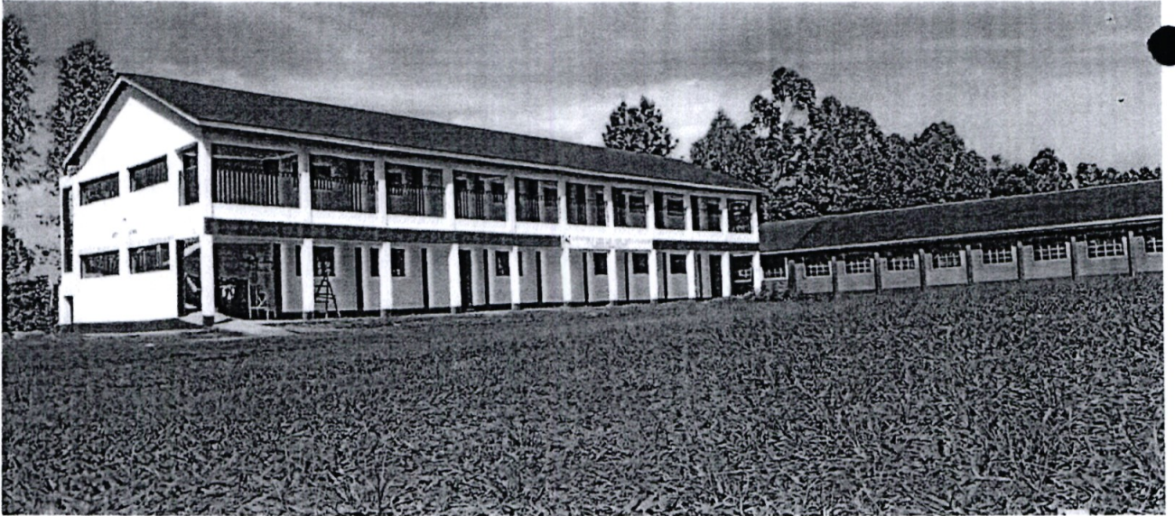
Construction of Twin Laboratory and 3 Classrooms at St. Maurice Mwira Secondary School
