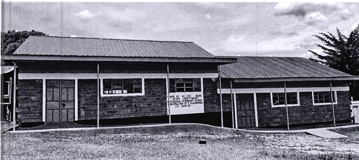
Mutarakwa Secondary School-Construction of 2 classrooms
