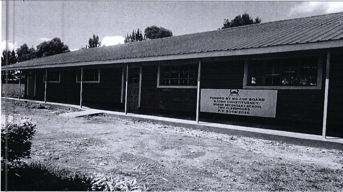
Ndege Secondary School- Construction of 2 classrooms
