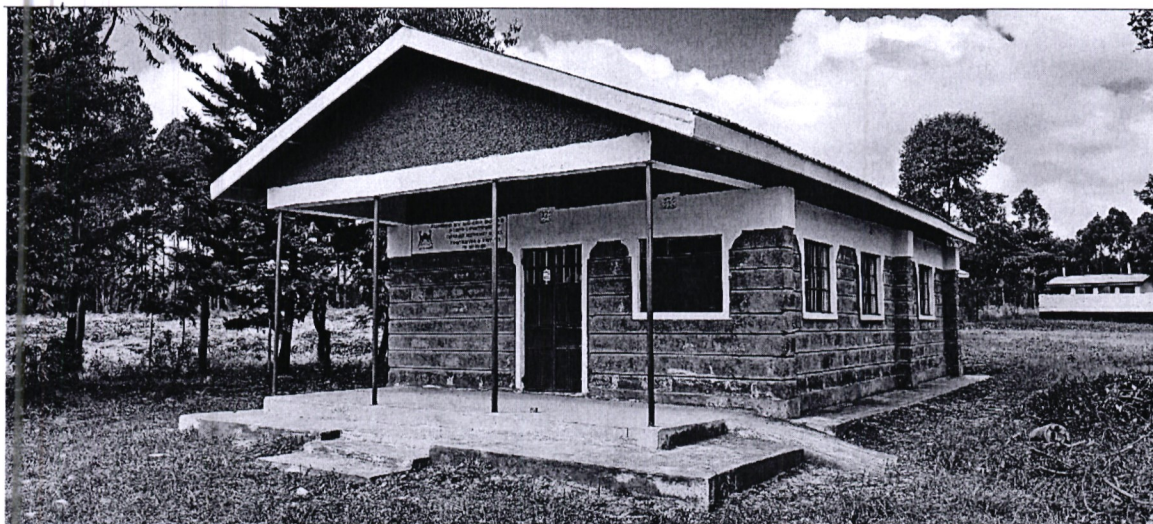
Tarakuet Secondary School- Construction of a Kitchen
