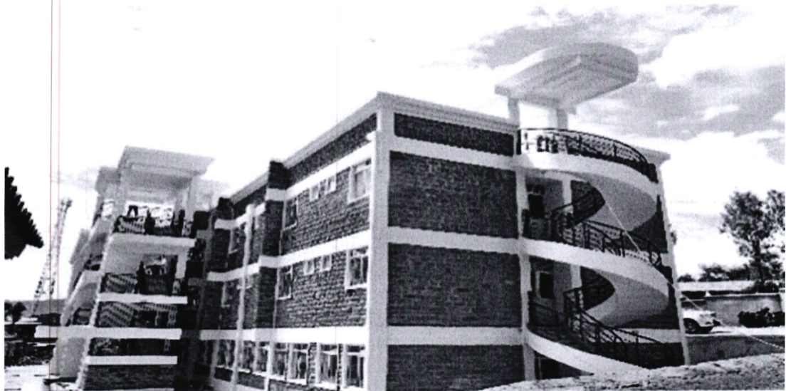
Figure 6: Marani Level 4 hospital in Kitutu Chache North Sub-County
