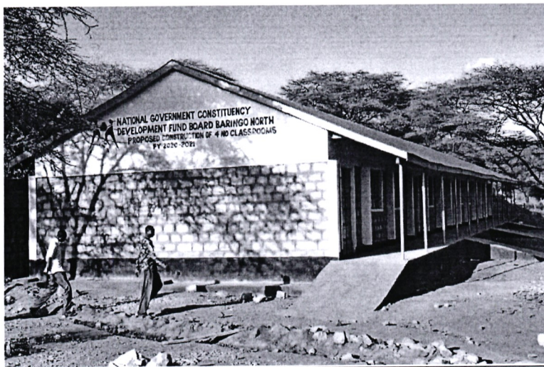
KAMPI NYAZI PRIMARY .CONSTRUCTION OF FOUR CLASSROOMS
