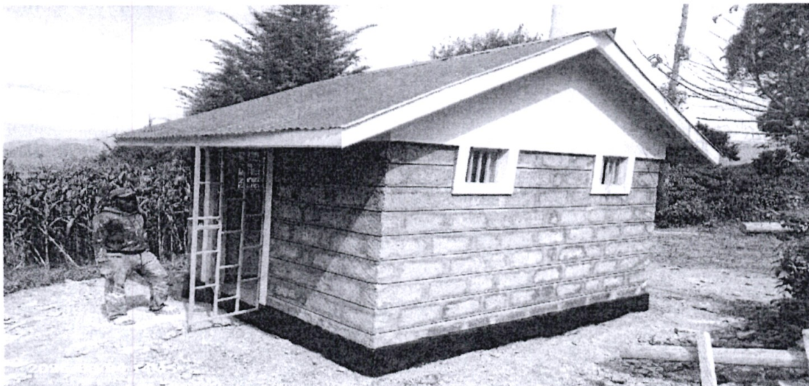
Ketigoi Asst Chiefs Office and Toilet Construction
