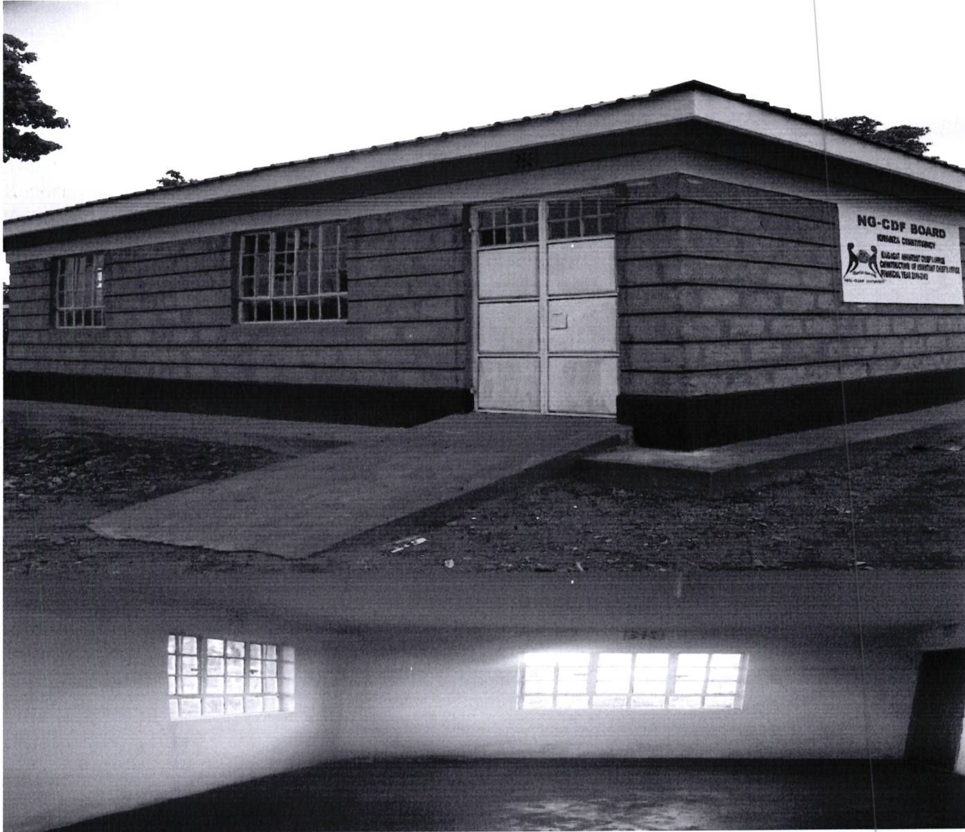
KAISAGAT ASSISTANT CHIEF'S OFFICE, CONSTRUCTION OF AN OFFICE-COMplete
