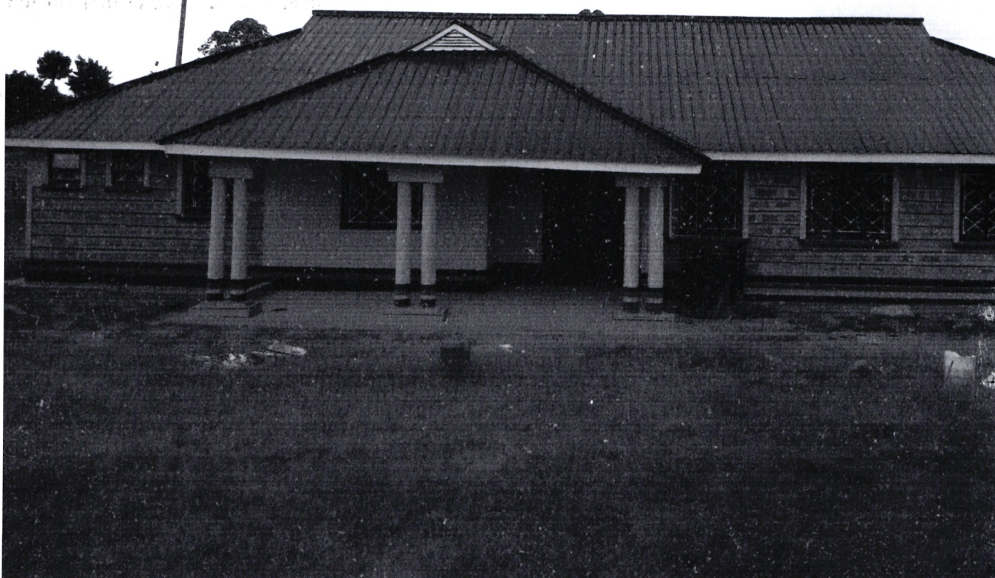
KWANZA OCPD, CONSTRUCTION OF OCPD'S OFFICE-COMLETE.
