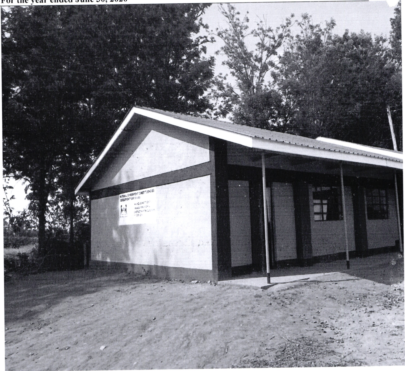
KWANUSU PRIMARY SCHOOL, CONSTRUCTION OF 2 CLASSROOMS-COMplete
