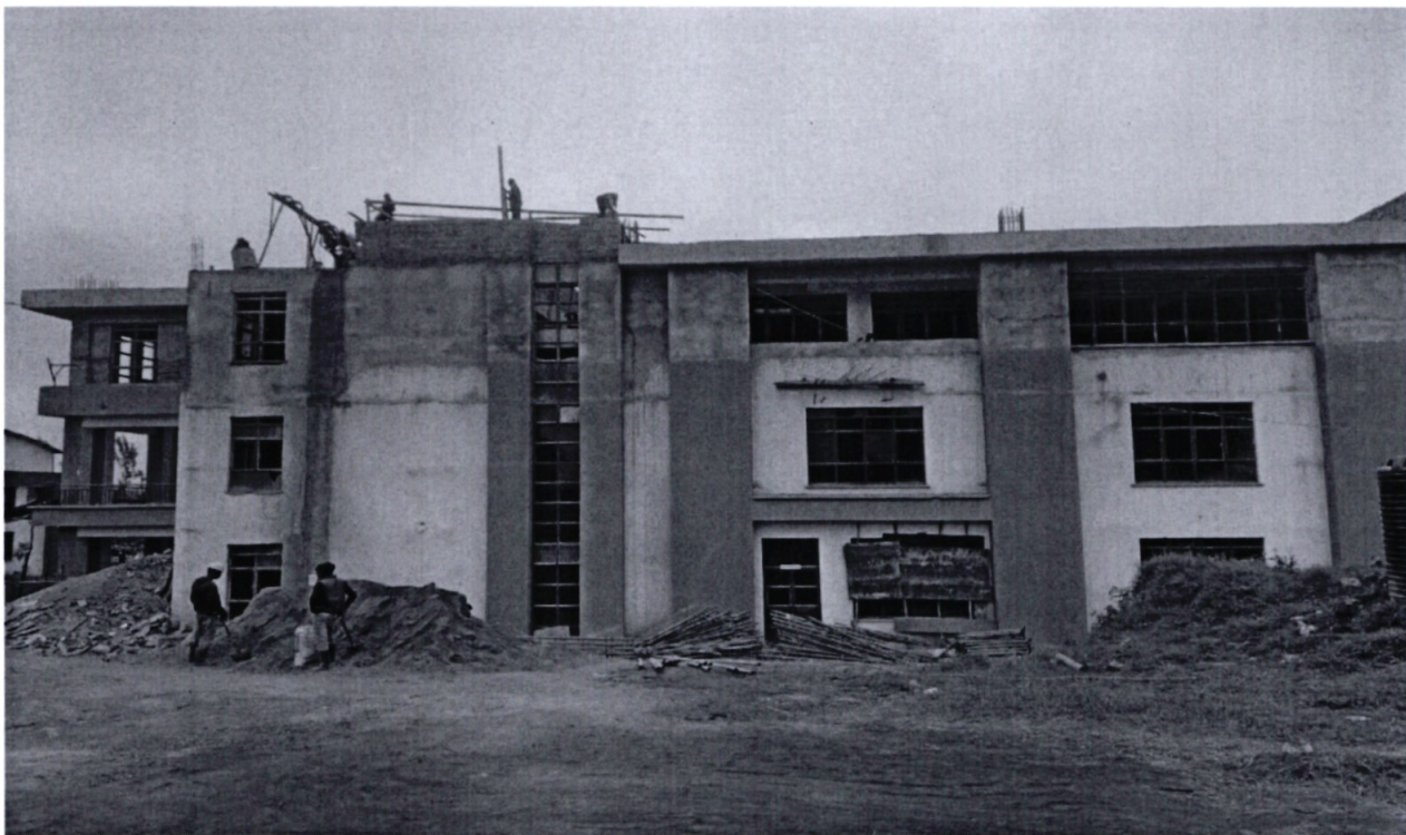
Tuition Block Phase II - ongoing
