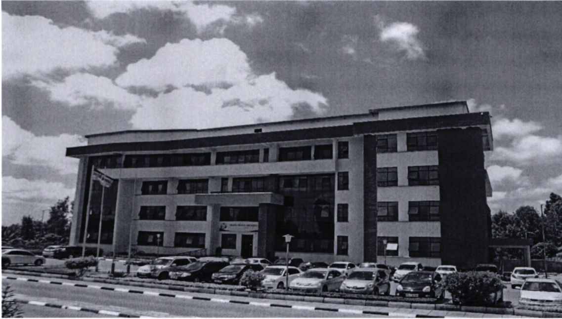
Administration Block – Awaiting final Accounts & Retention Refund
