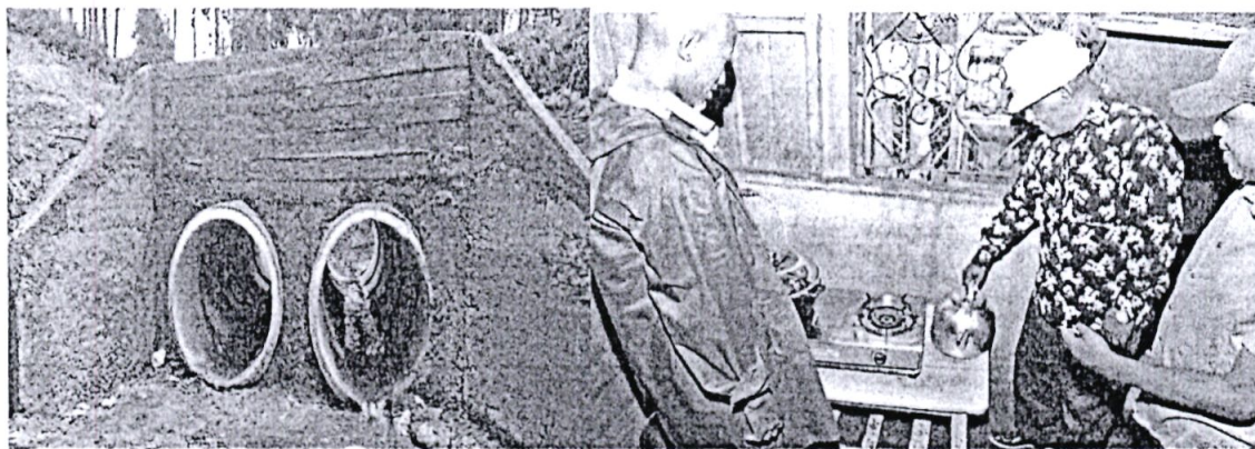
Mere, Kabaru ward Double box culvert bridge under construction H.E, the Governor checking a biogas project in Kangaita Aguthi, Tetu
