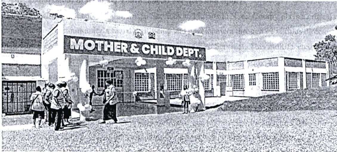
The new mother and child Hospital at the Nyeri Health Centre at Nyeri Town
