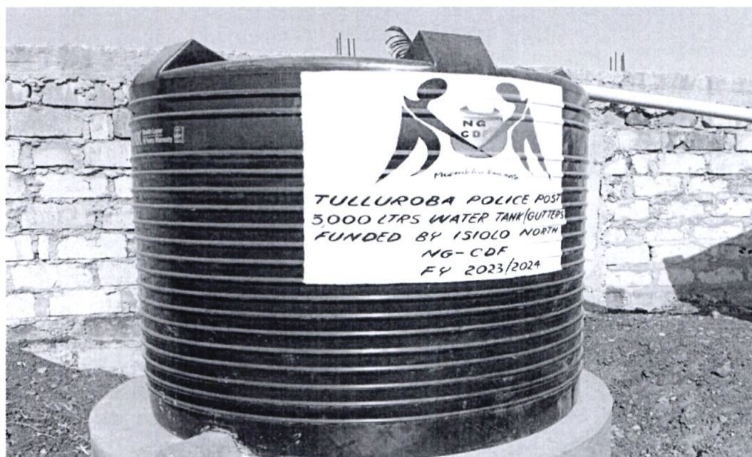
Climate Change Project-Installation of water tank at Tullu Roba Police post.
