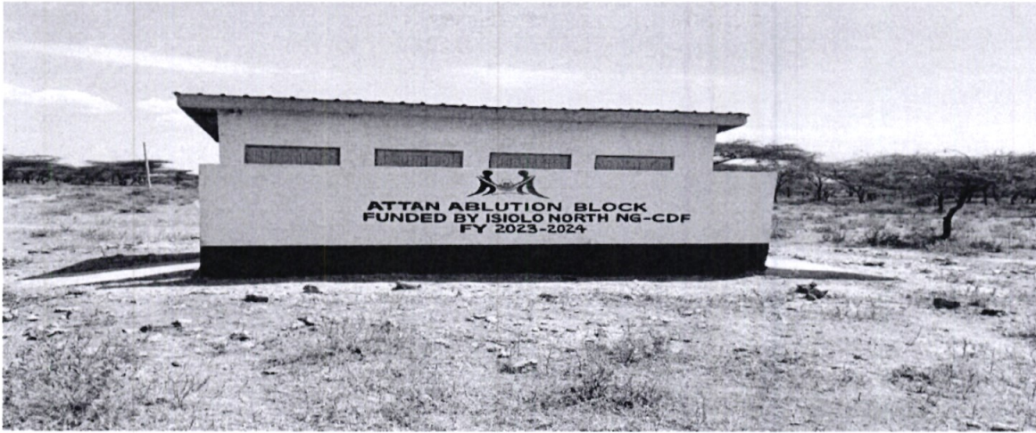
ATTAN CHIEFS OFFICE –TOILETS
