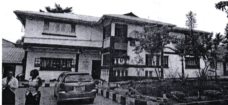
The Administration block at Nyaikuro secondary school funded Kshs. 500,000 2016/2017FY
