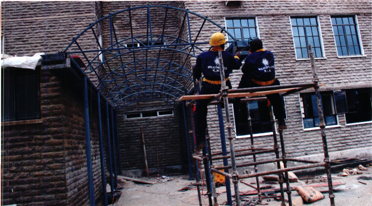
Maintenance work at County Hall
