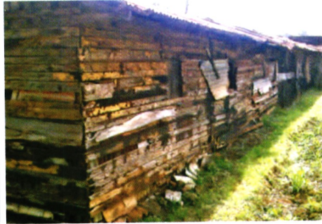
Police accommodation at Kerugoya Police station
