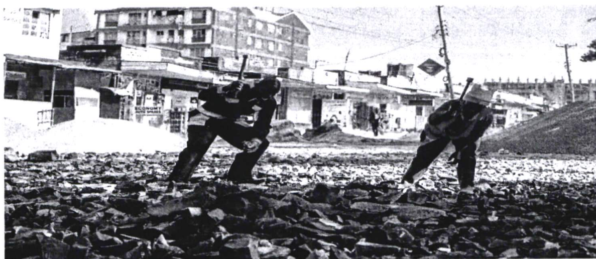
Ongoing rehabilitation of roads
