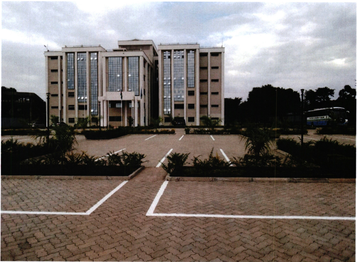
Administration and Lecture Halls Block Phase I Completed
