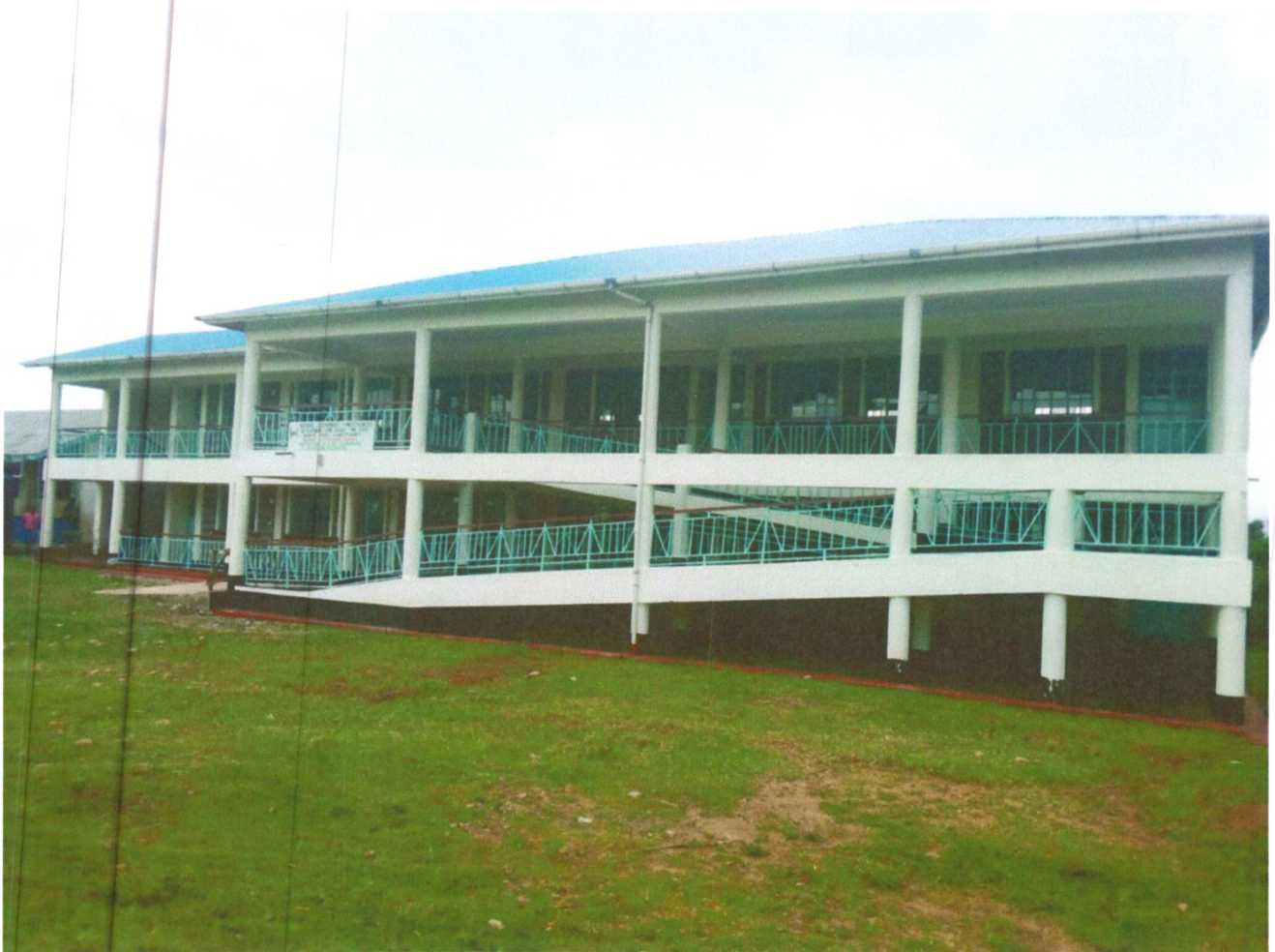
Picture-1 Lugulu day Secondary School Webuye West- Six classrooms storey block with ramp
