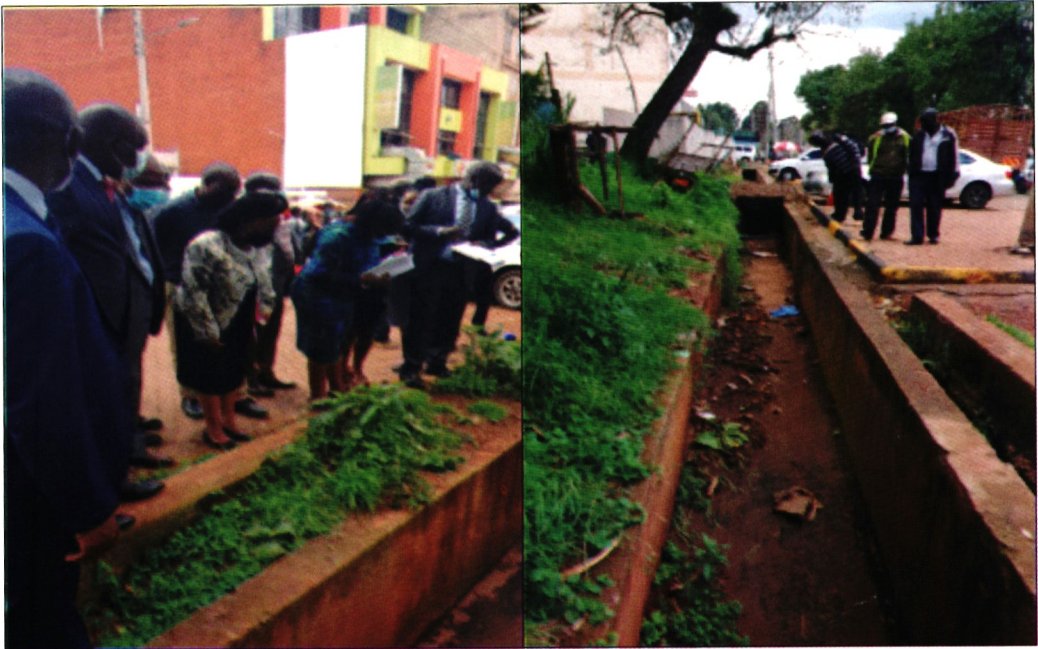
Figure 4: Construction of stormwater drainage facility-Kericho County
