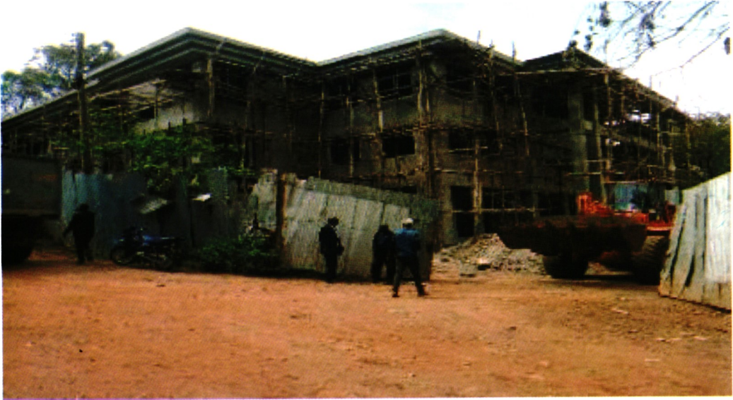
Figure 3: Constructions of County Assembly Chambers -Marsabit County
