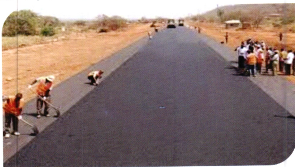
Figure 22: Construction of the Kibwezi- Mutomo- Kitui Highway
