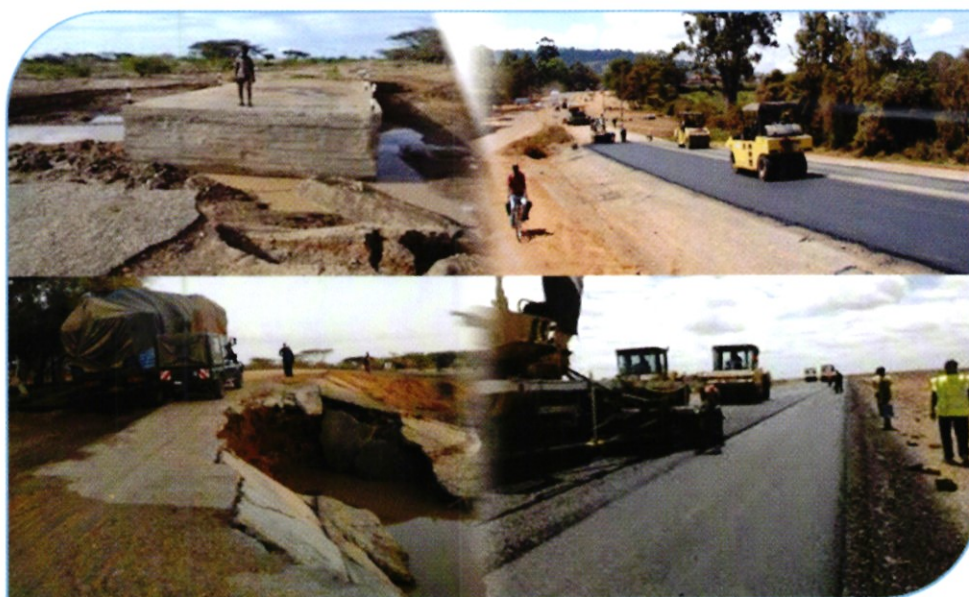
Figure 21: Rehabilitation of key infrastructure
