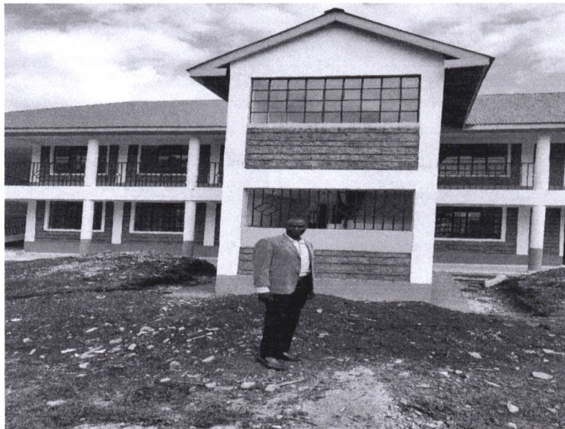
Photo: Bomachoge Chache KMTTC Project, Ongoing Phase II
