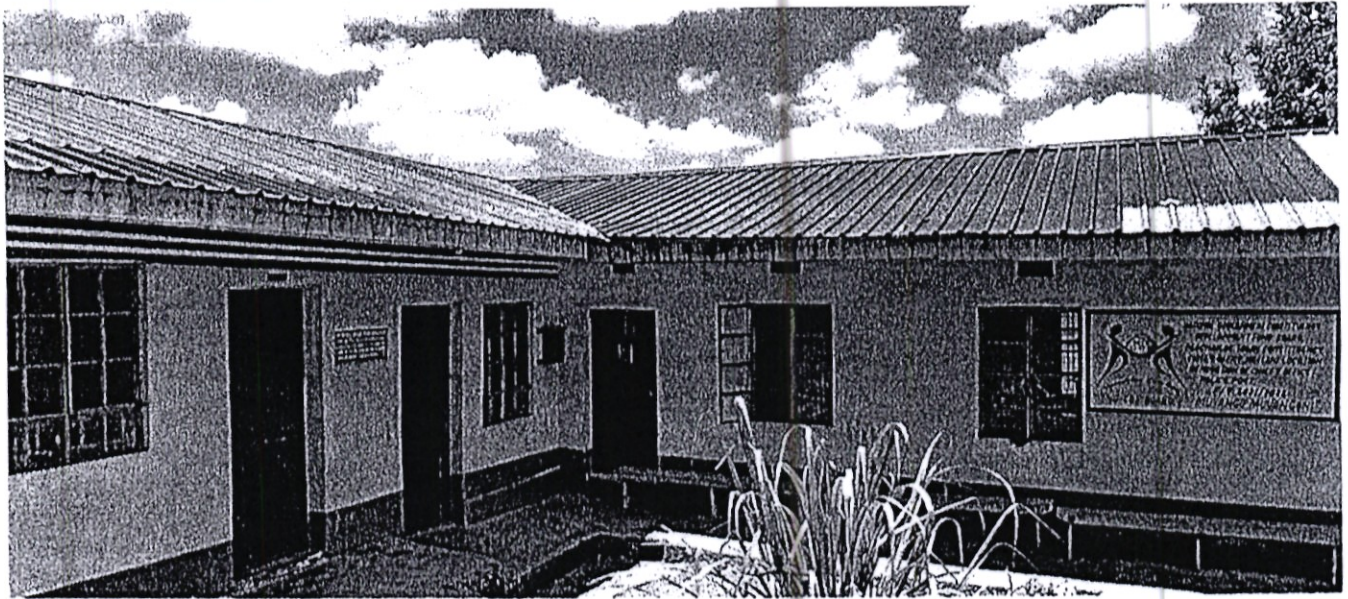
Ngelani Chiefs office- Renovation of 5 roomed chiefs office / police post Ksh 700,000
