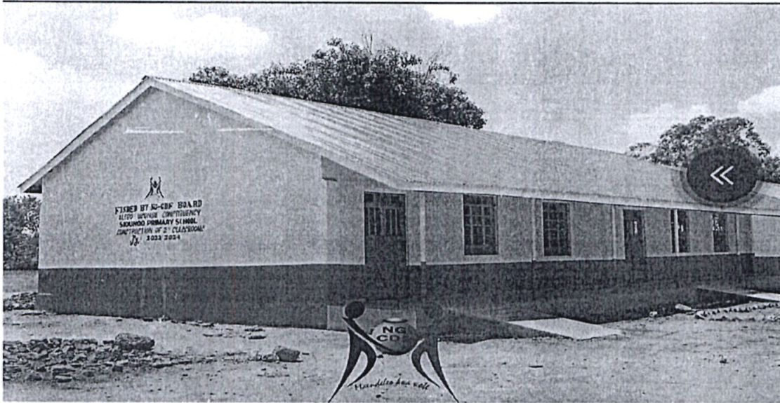
Project 1: Sidundo Primary school: renovation of 2 No classrooms
