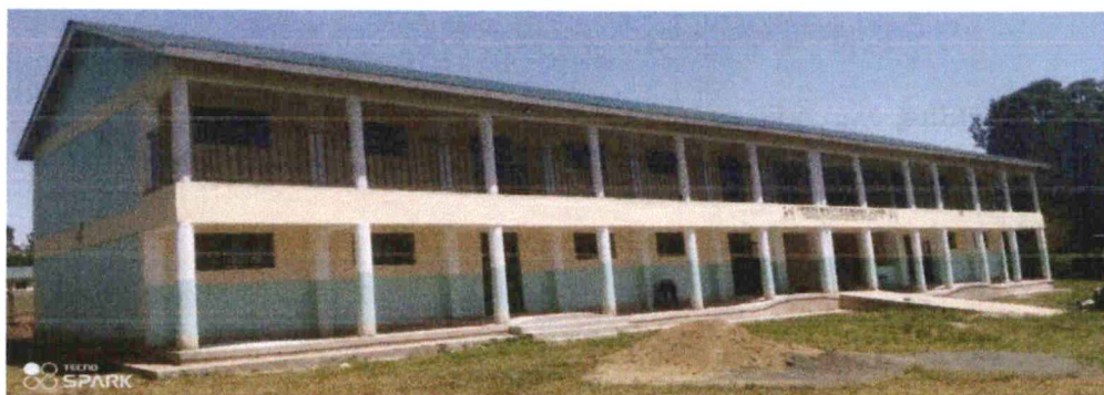
Emwiru Mixed Secondary School - Construction of 6no.classrooms.
