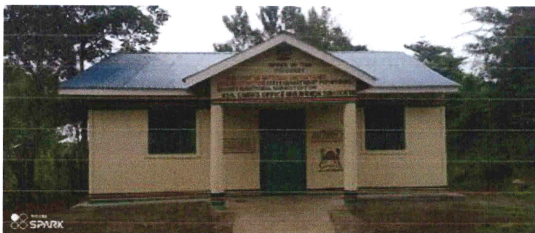
Assistant Chief's Office, Mulwanda – Construction of an Administration block. -Complete, handed over and in use. This provides a conducive working environment to the administration as they serve the constituents.
