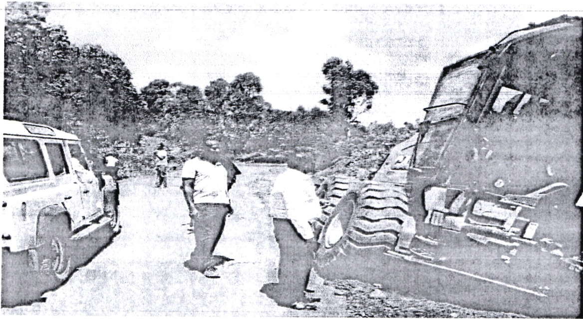
The road leading to Dudi Girls' Secondary School being graded.
