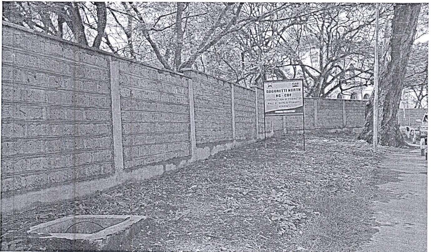
Figure 1: Construction of a Perimeter wall at Nairobi Primary School.
