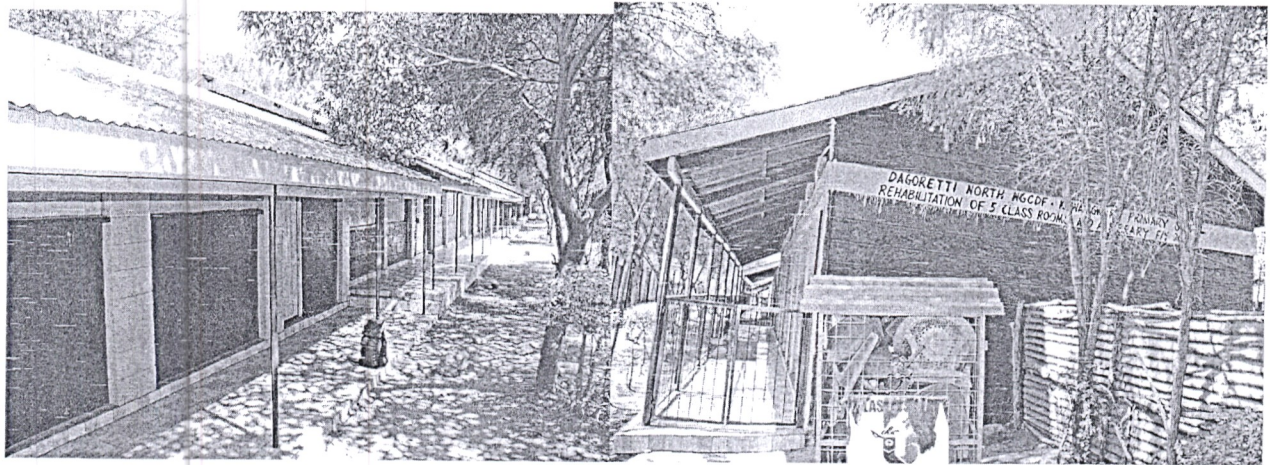
Figure 4: Renovation of Classrooms at Kawangware Primary School
