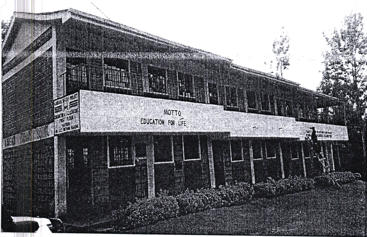
Muri-ini Day Secondary School Classroom Block
