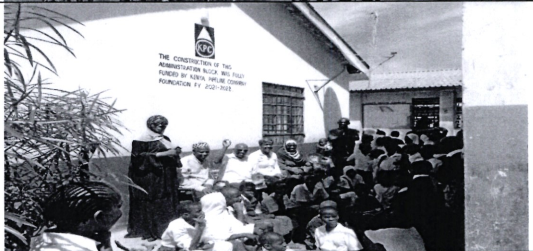
KPC Foundation sponsored the construction of an administration block at a cost of Kshs. 4Million at Kwahola Primary school in Mombasa County.
