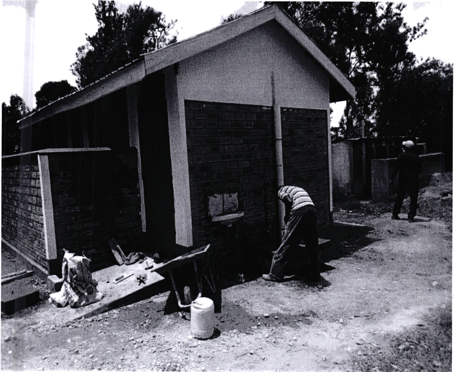
Project Name: Ruambwa Primary school Activity: Construction of a 12-door modern flash toilet with a solar pump water supply.
