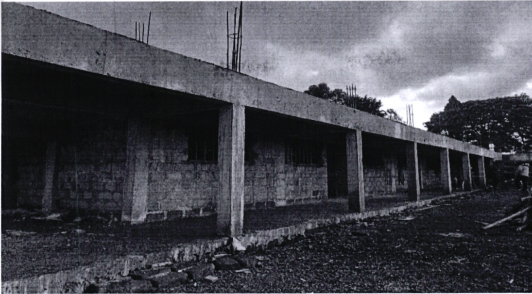
Ongoing Construction of 18 number classrooms at Nyamira Comprehensive School
