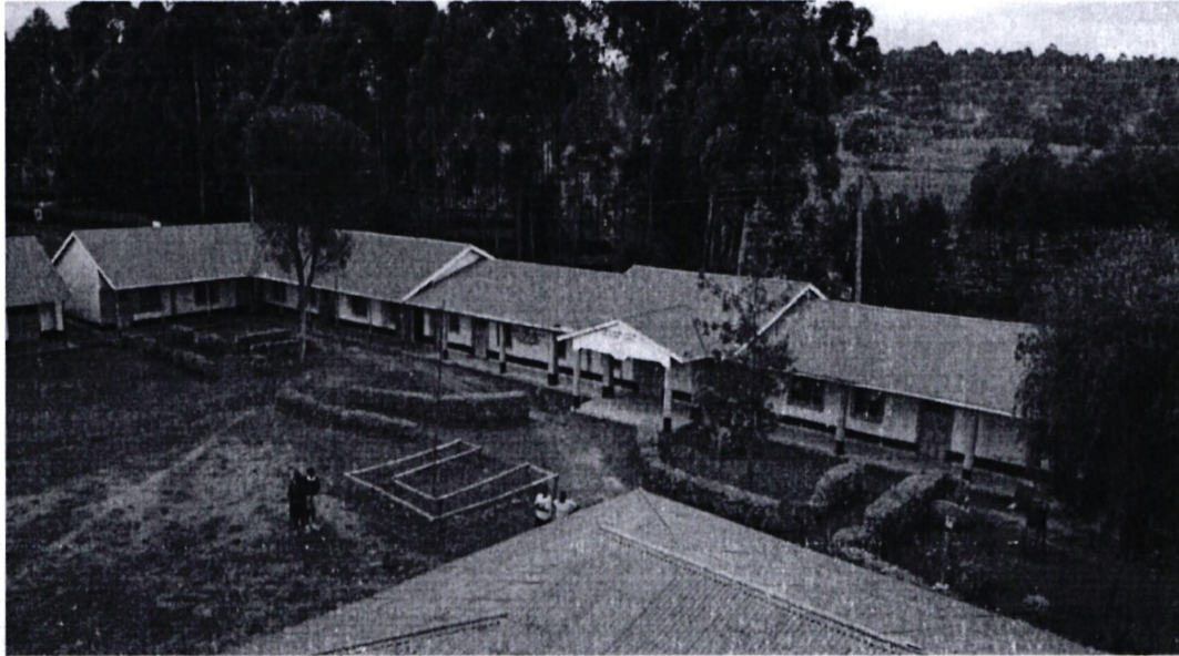
EKENYORO TECH. MIXED SEC SCHOOL. Renovation of 8 no. classrooms
