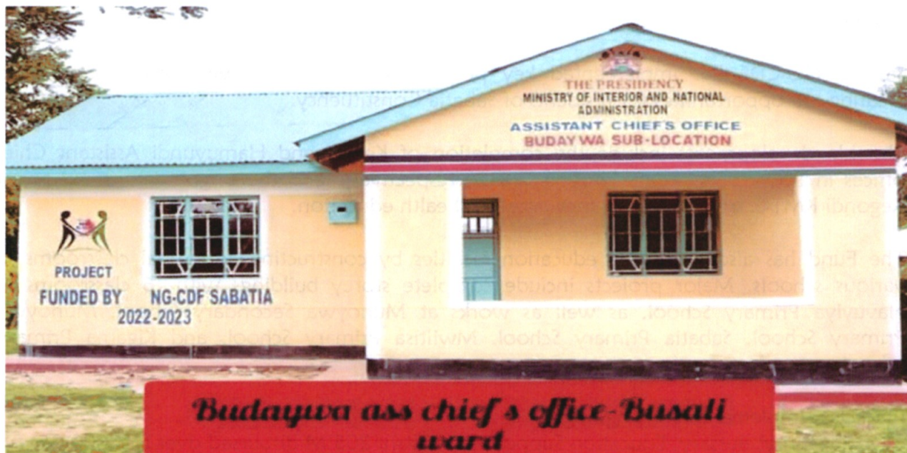
Image Showing the complete construction of Assistant Chief office at Budaywa Asst Chief office
