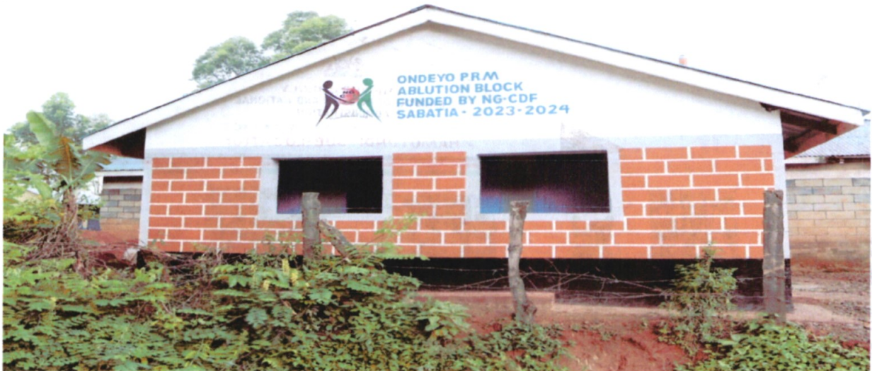
Image 4: Complete construction of an abulation Pit Latrine at Ondeyo Primary School
