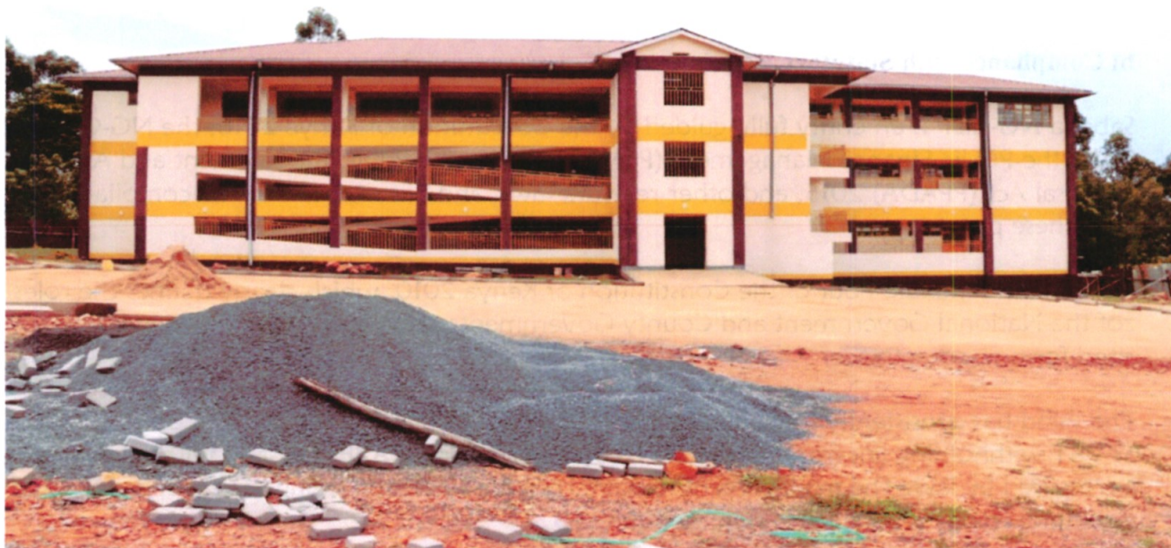
Image Showing the construction at Kegondi KMTC
