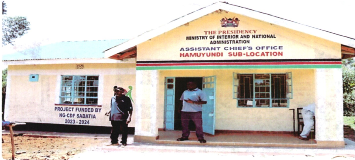
Image 2: Complete Construction of Hamuyundi ast chief office
