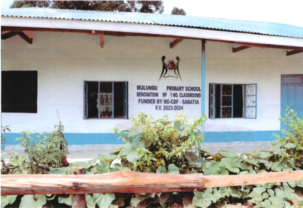
Image 1: Complete Renovation of 1No. Classroom at Mulundu Primary School.
