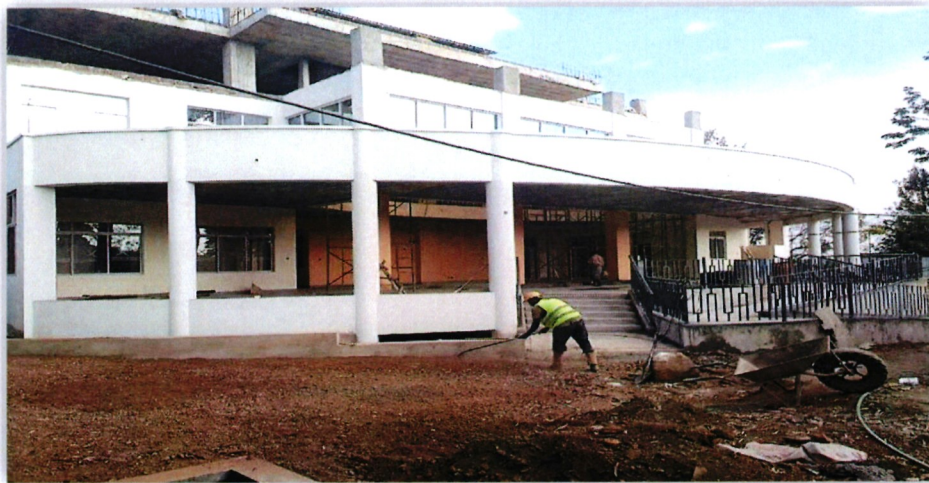
Ongoing works at KNH Cancer Center
