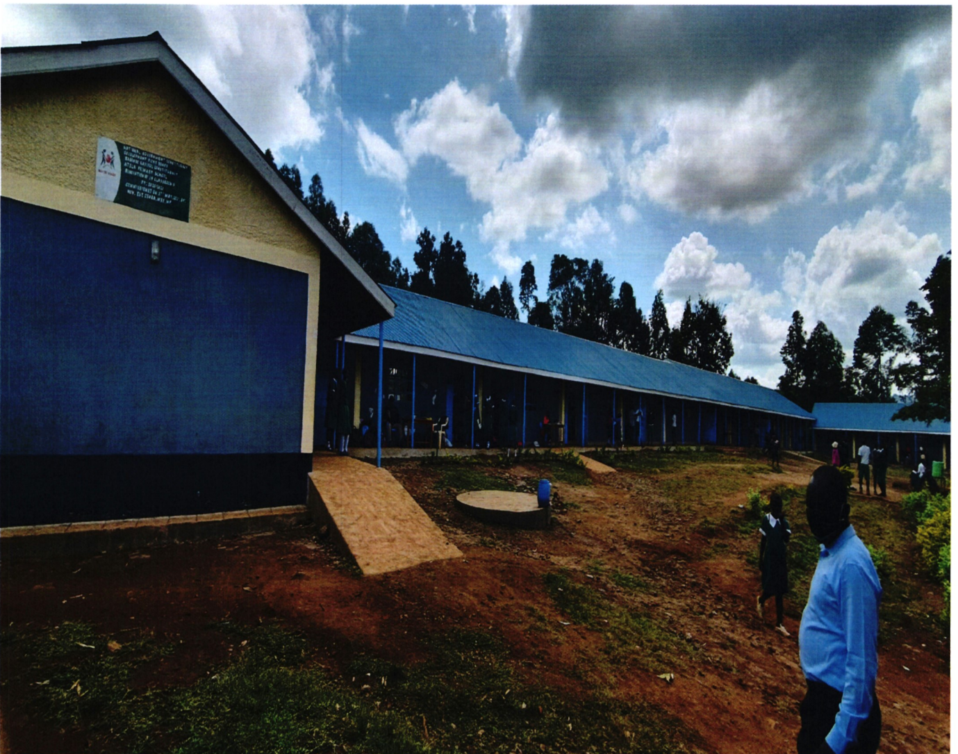
Fig 2 b: Atela Primary School: Rehabilitation of 14 Classrooms
