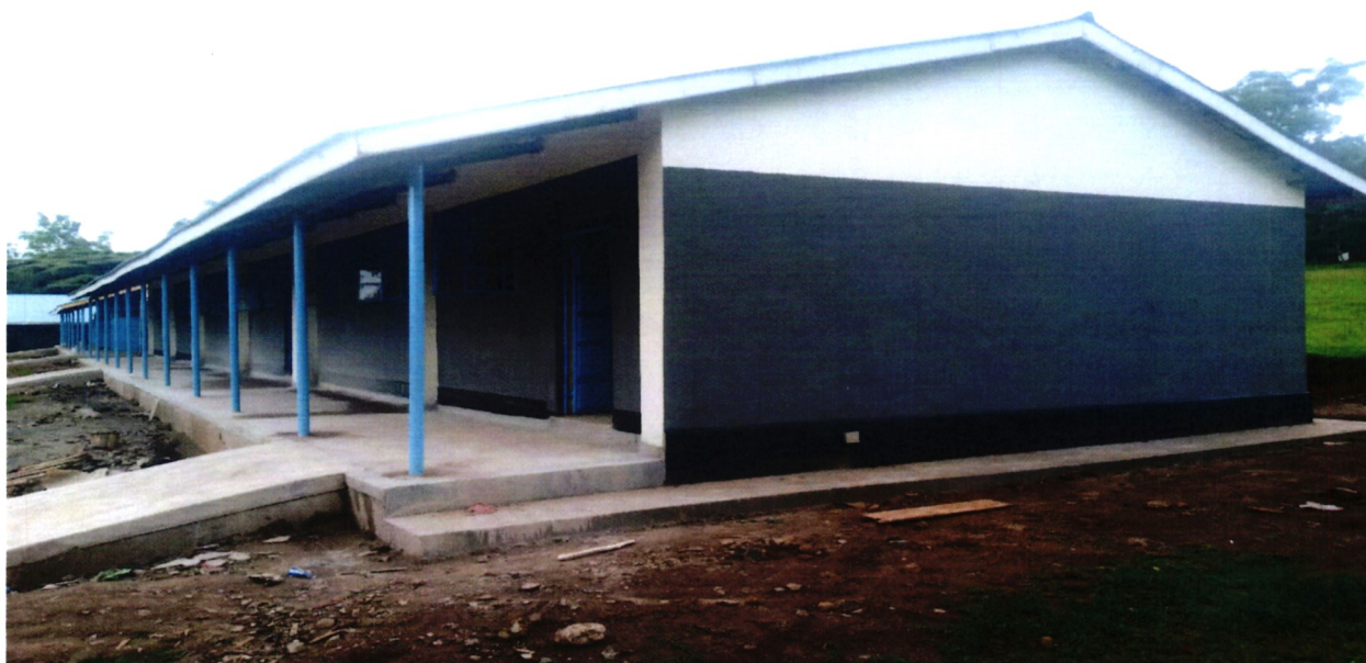
Fig 3: Dudi Primary School: Renovation of 11 classrooms
