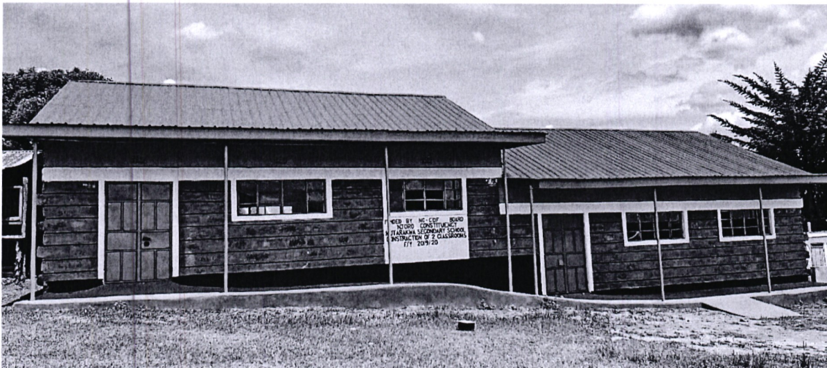
Mutarakwa Secondary School-Construction of 2 classrooms
