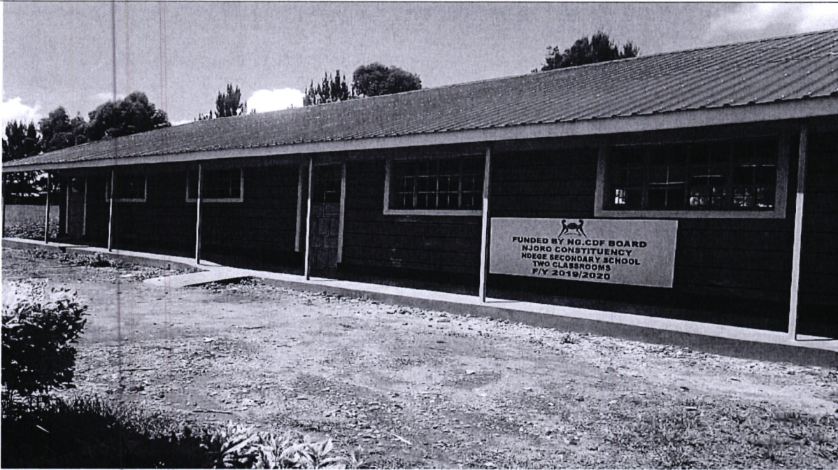
Ndege Secondary School- Construction of 2 classrooms
