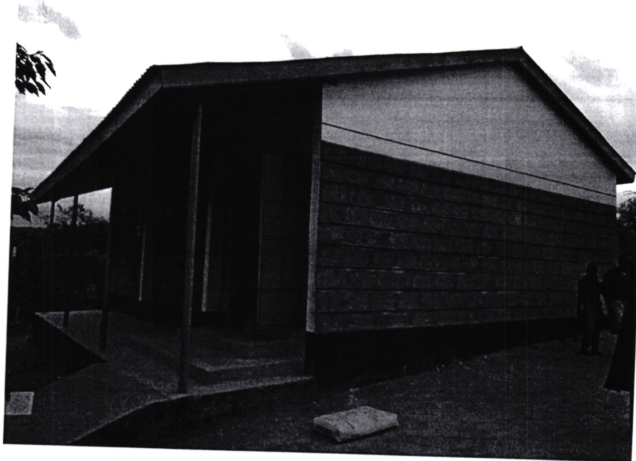
FIG 6 MULANG'A PRIMARY SCHOOL COMPLETE CONSTRUCTION OF CLASSROOM.
