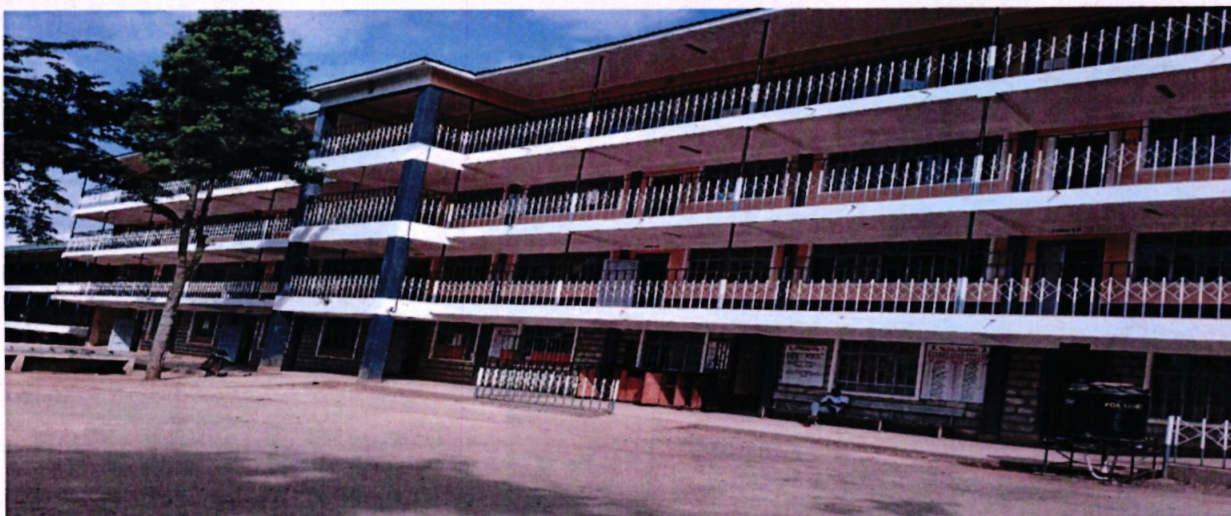
Meru high school: construction to completion of tuition block
