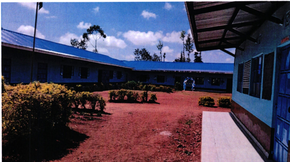
Kiamiriru Primary school; fully renovated: reroofed tiled and repainted in 2024-2025
