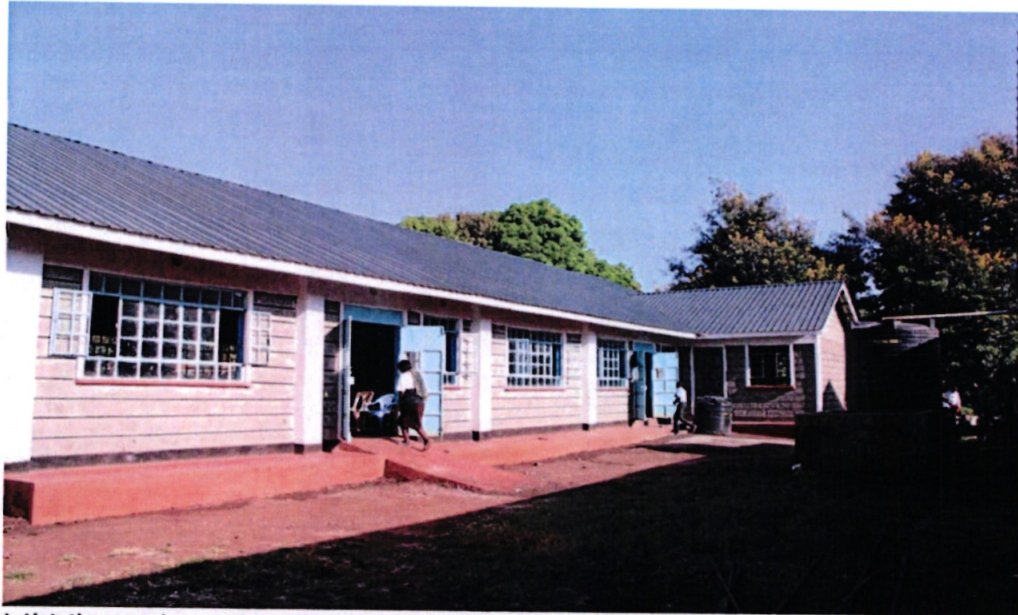
Mbirikene day secondary school- construction to completion of dining hall
